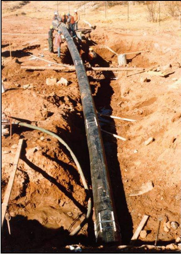
Figure B-69. —Inserting the HDPE slipliner into the existing CMP conduit.
