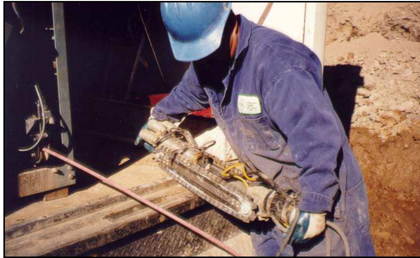
Figure 130. —Most CCTV inspection equipment is portable and can be carried to conduit access locations.
