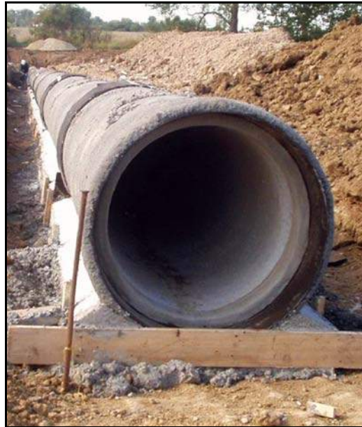
Figure 60. —Precast concrete using bedding as support.
