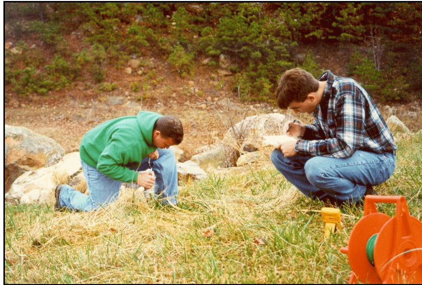
Figure 141. —Collecting self potential (SP) data on the crest of an embankment dam in Virginia to trace the source of observed seepage. The 75-ft high embankment dam had a sinkhole, a sand boil, and several seepage points on the downstream face. This information was used in complement with electrical resistivity imaging data. Photo courtesy Schnabel Engineering.
