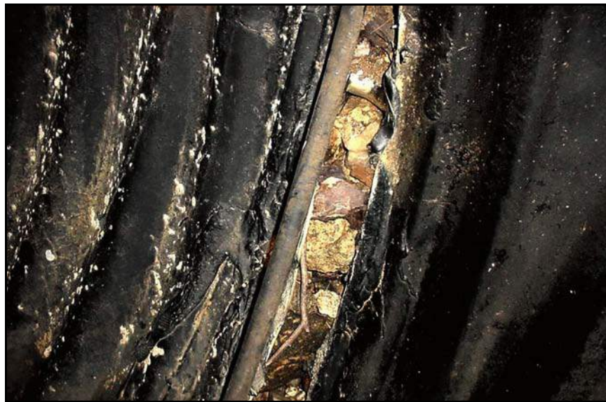
Figure B-52. —The failed embankment dam was repaired with a new 78-in diameter CMP spillway. However, soon after reconstruction, this failed joint was discovered at the upstream end of the pipe near the riser. A large void was also observed in the adjacent embankment fill. Note the o-ring gasket has been displaced from the joint.
