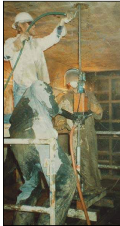
Figure B-45. —Grouting operations within the conduit.
