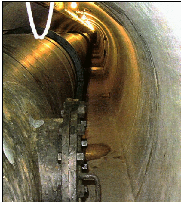
Figure 55. —An example of the interior of conduit shape B.
