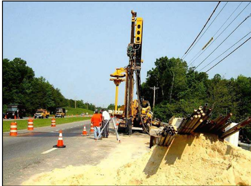
Figure B-32. —The failed CMP and voids were filled with a stiff compaction grout.
