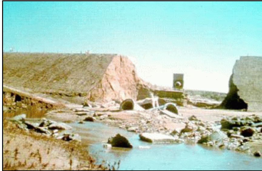
Figure 6. —Embankment dam failure caused by internal erosion of earthfill near the conduit. The initial failure was tunnel shaped, but the collapse of the roof of the tunnel resulted in the observed shape of breach. Hydraulic fracture in highly dispersive clay embankment soils caused the failure. The embankment dam design included antiseep collars, but no filter diaphragm.
