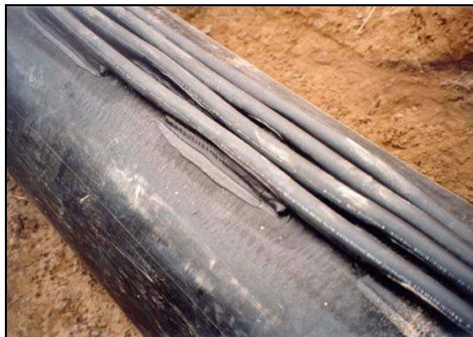
Figure 168.—HDPE grout pipe attached to HDPE slipliner.
