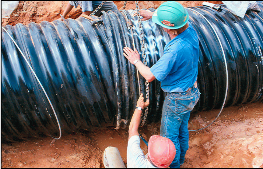
Figure 31. —A CMP conduit being installed.
