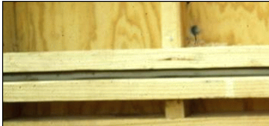
Figure 78. —Waterstop held firmly in place by use of a specially cut slot in the form.
