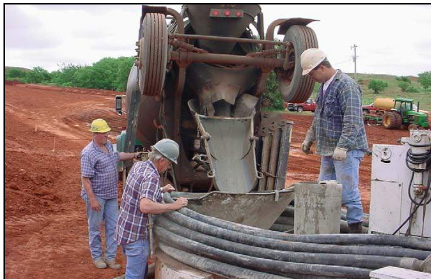
Figure 200. —Grout being delivered to the pumping truck.
