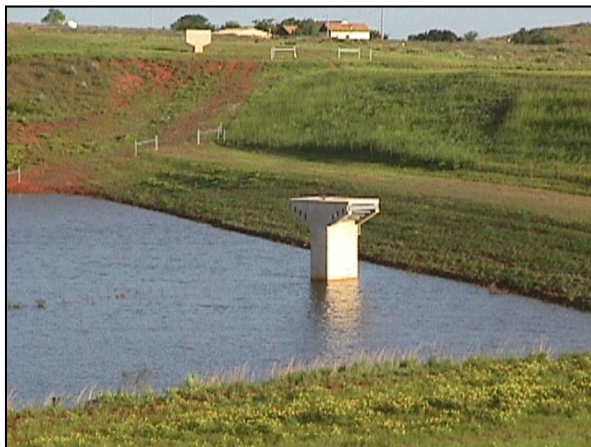
Figure 40. —The riser structure for a principal spillway.
