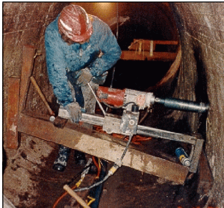
Figure 191. —Drilling a grout hole from the interior of a conduit.
