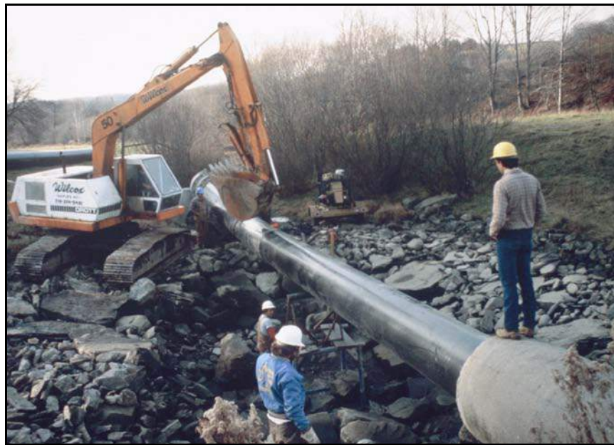
Figure 171. —Insertion of an HDPE slipliner into an existing concrete conduit. A backhoe is being used to assist with slipliner insertion.
