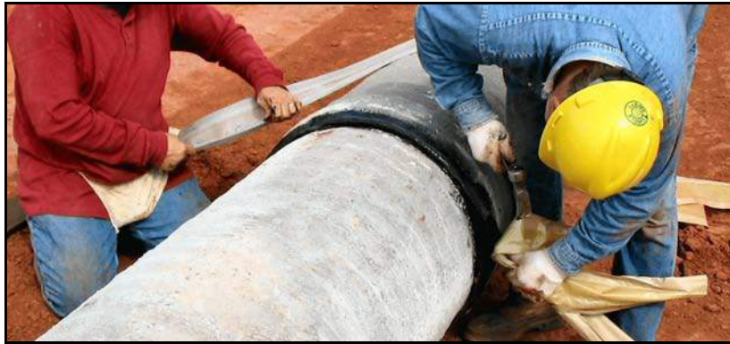
Figure 80. —Mastic being applied to exterior annular joint space of precast concrete pipe.
