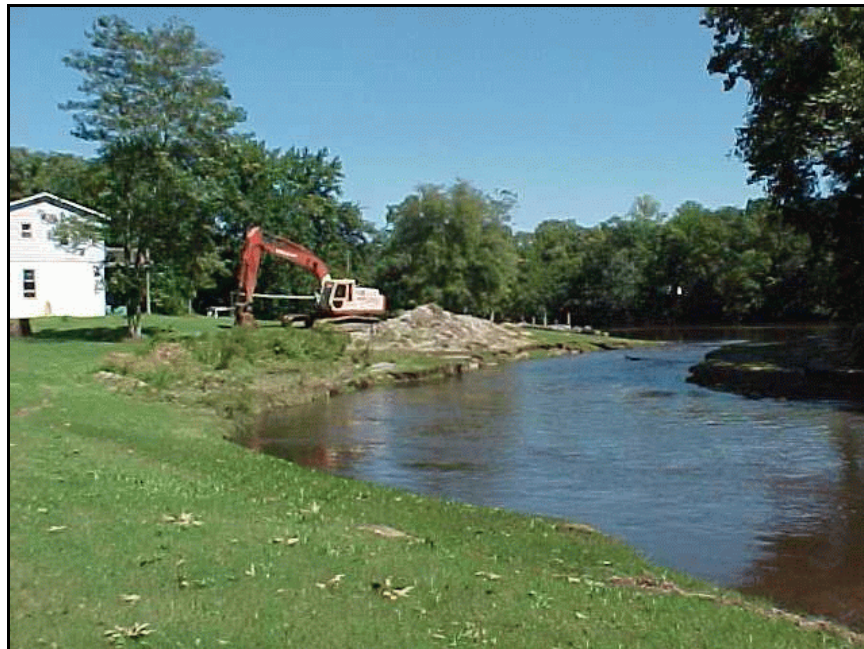
Figure 156. —The owner of this embankment dam excavated a channel around the dam to prevent its overtopping during a hurricane.
