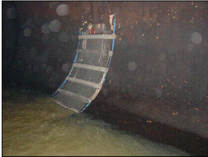
Figure B-14. —Metal plate bolted across the joint.
