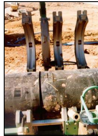
Figure 164. —Finished fusion welded joint.
