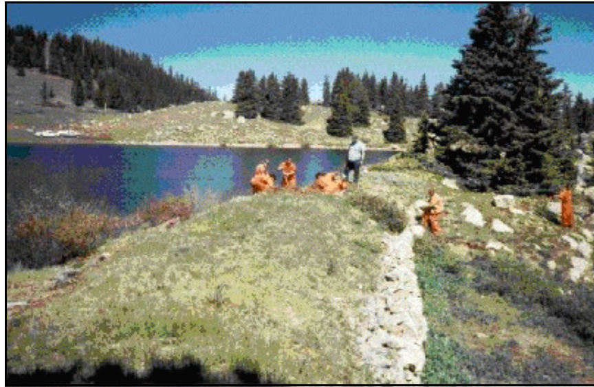
Figure B-38. —Excavation of the controlled breach in the embankment dam.
