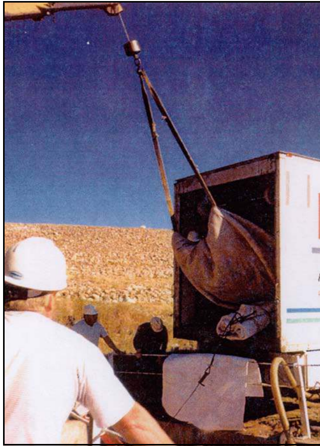
Figure B-80. —Lowering of the CIPP liner into the stilling basin, so it can be winched up the tunnel.
