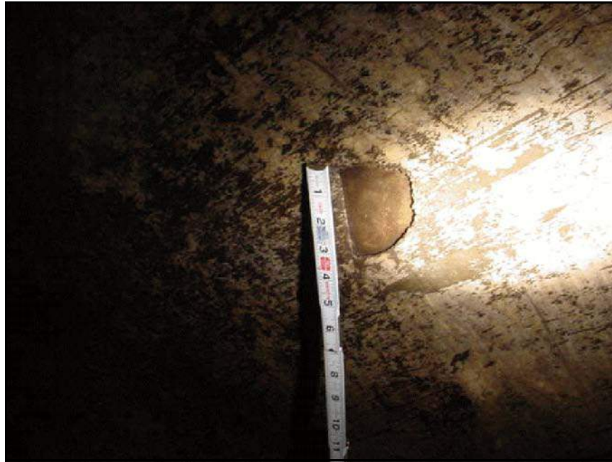
Figure B-22. —Popout located at station 10+79.
