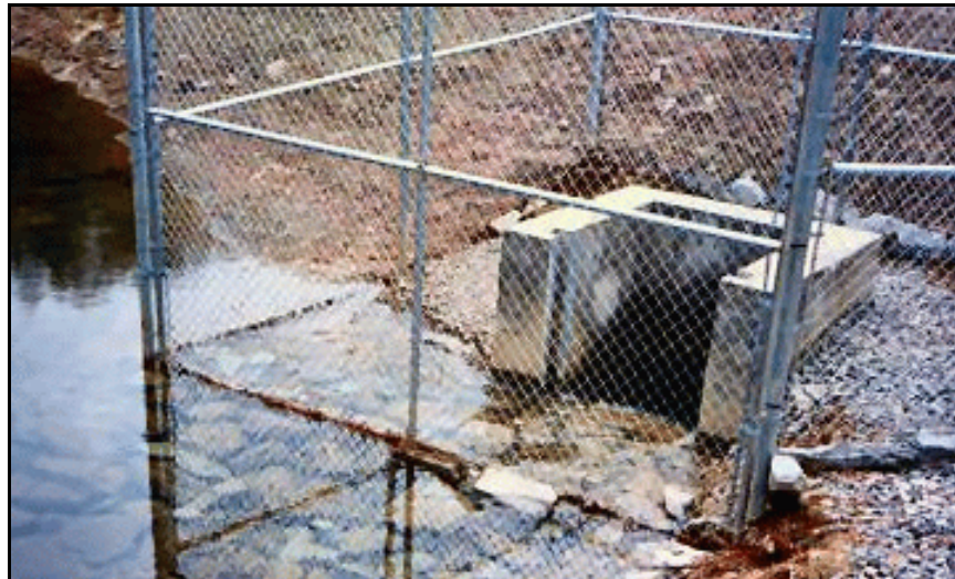
Figure 13. —An example of a decant intake structure.
