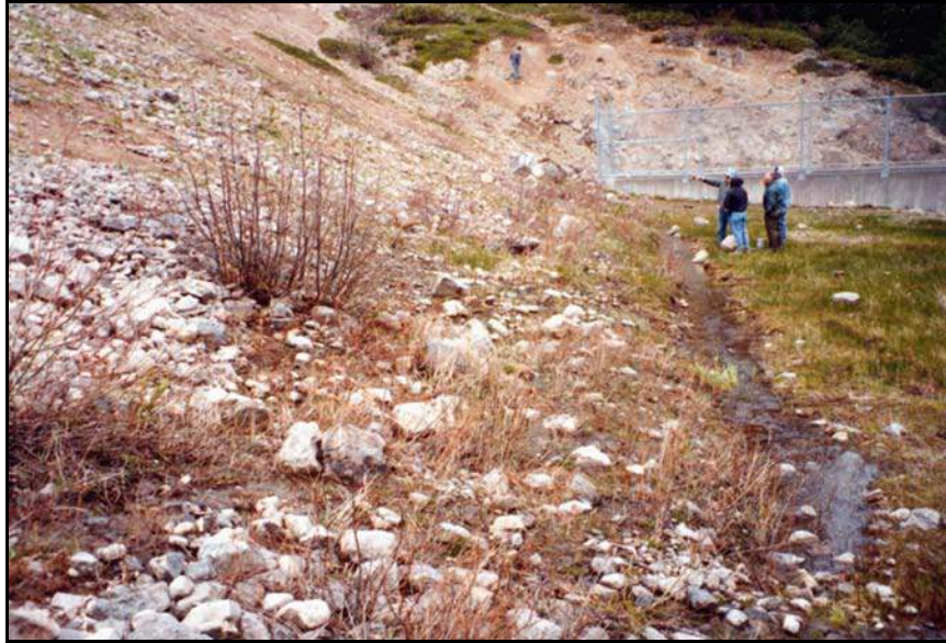
Figure 118. —Visual inspection for seepage on the downstream face of an embankment dam.
