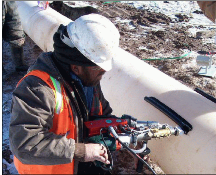
Figure 169. —Spacers being attached to an HDPE slipliner using an extrusion gun.
