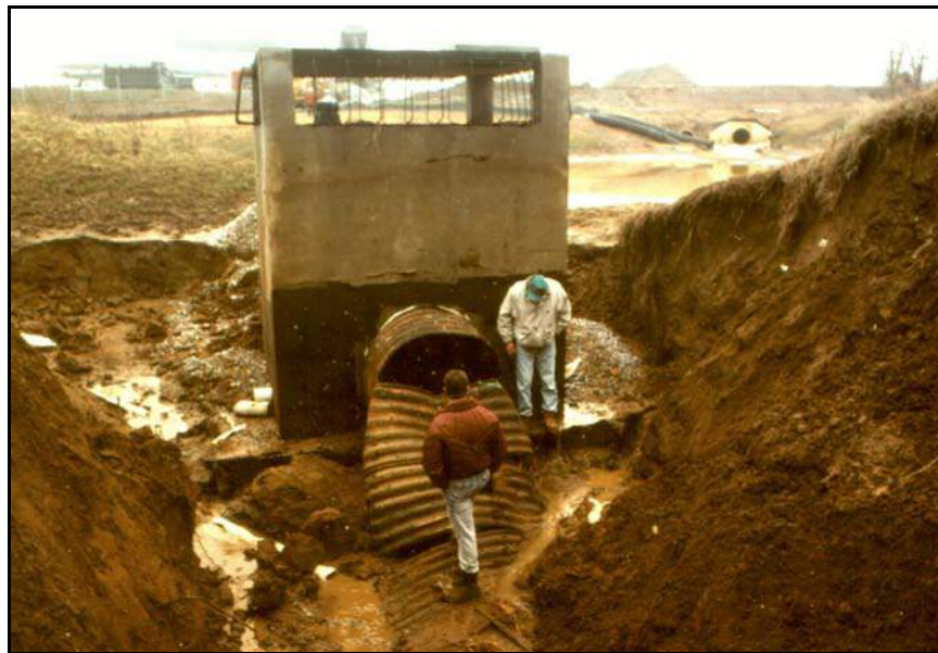
Figure B-5. —The upstream section of the 54-inch diameter CMP spillway conduit completely collapsed when the water level reached the elevation of the weirs on the inlet structure. Site personnel reported a “vortex” in the pool adjacent to the structure shortly before collapse.
