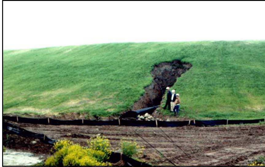
Figure B-55. —When the pool level of this embankment dam was only about 2 to 3 feet deep, flow along the outside of the CMP resulted in loss of the adjacent soils.
