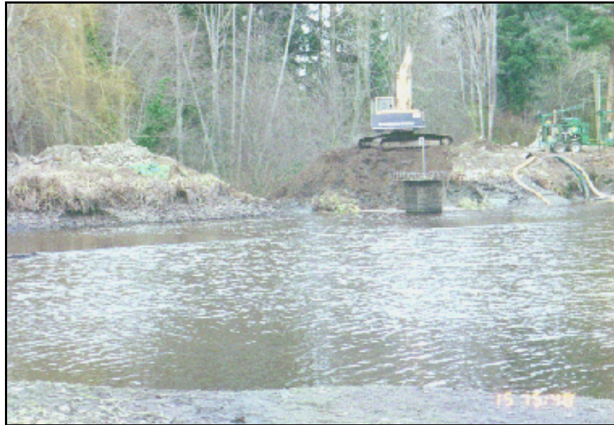
Figure B-57. —View of upstream dam crest nearing completion of breach.
