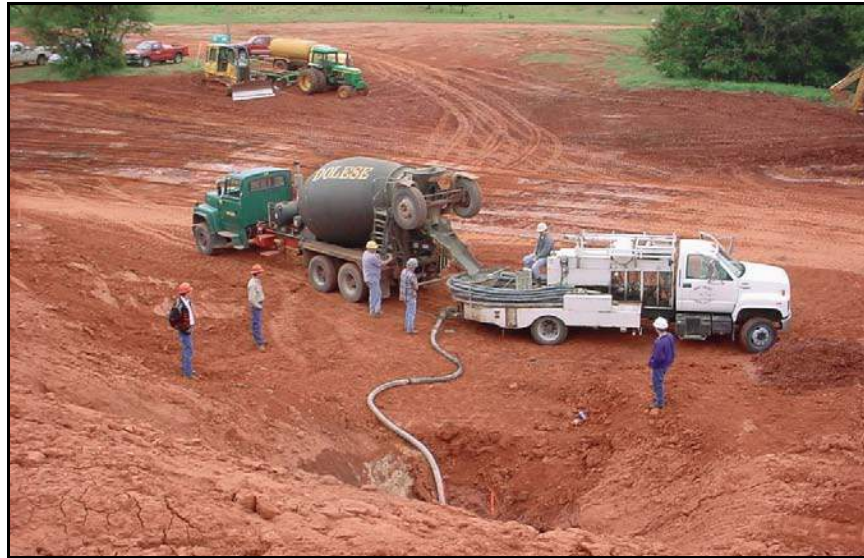
Figure 199. —Grout is delivered to the site and is pumped into the conduit being abandoned.
