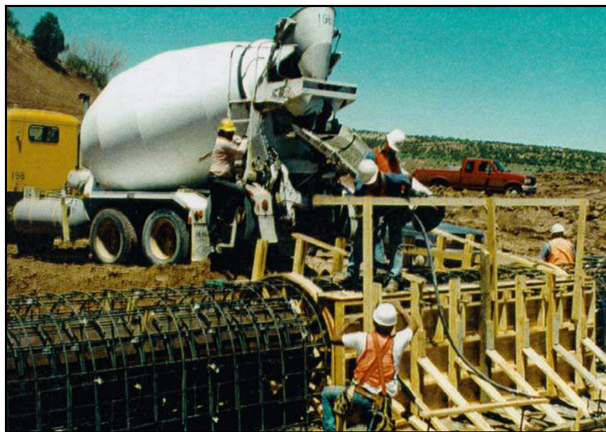
Figure 22. —Concrete placement for a reinforced cast-in-place conduit.
