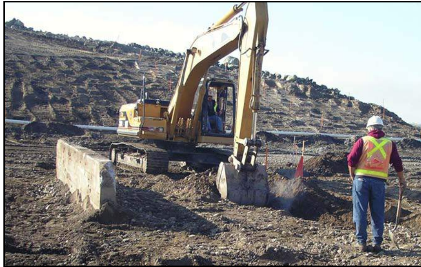
Figure 135. —An outlet works conduit is being excavated during a forensic investigation. The top of an antiseep collar is exposed on the left side of the figure.
