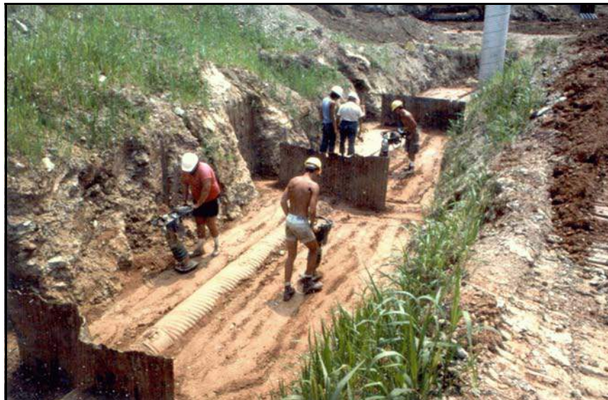
Figure B-54. —The embankment dam was constructed with antiseep collars.
