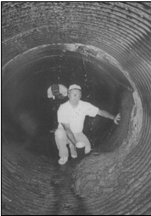
Figure B-36. —A man-entry inspection of this 60-inch CMP noted seepage and extensive loss of embankment soil at two locations.
