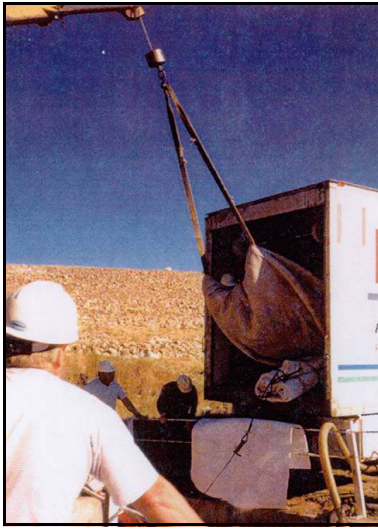
Figure 182. —Unloading the CIPP liner prior to installation.
