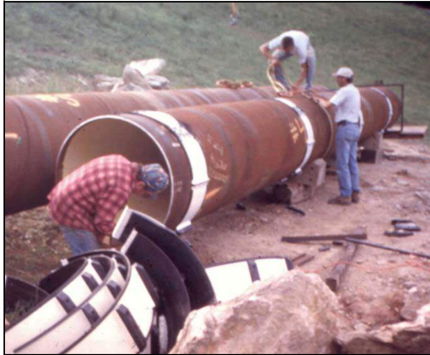
Figure 181. —Spacers being installed on a steel pipe slipliner.
