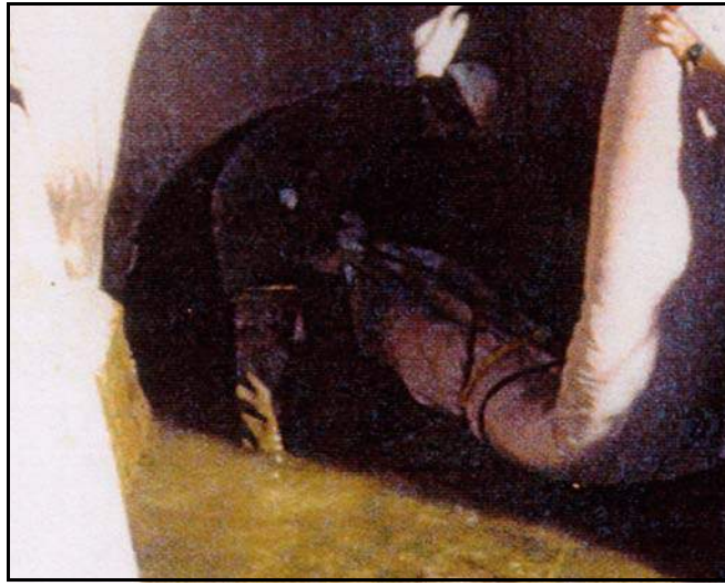
Figure 183. —CIPP liner being positioned for installation.
