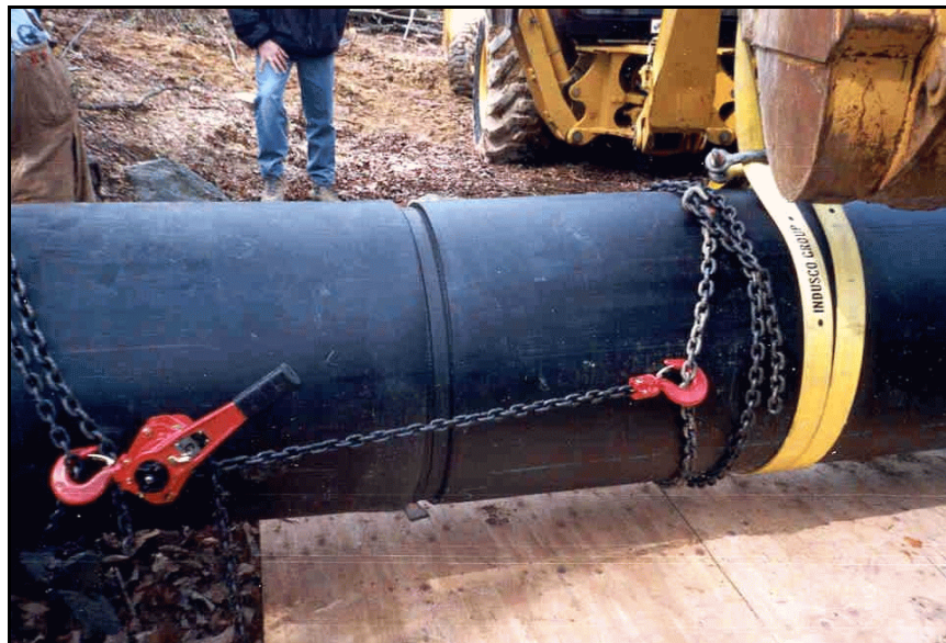
Figure 179. —Sections of proprietary Snap-Tite® pipe can be easily handled with small equipment.
