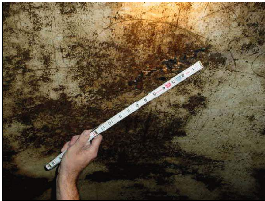
Figure B-21. —Exposed aggregate located at station 11+28.
