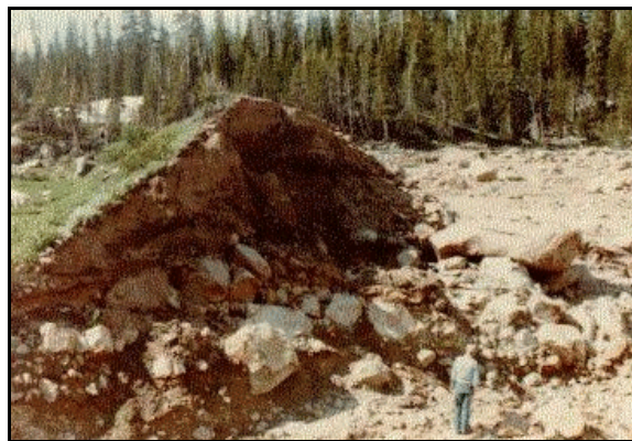
Figure B-47. —Right side of the breached Lawn Lake Dam.
