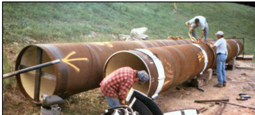
Figure 27. —Steel pipe slipliner being prepared for insertion into an existing conduit.
