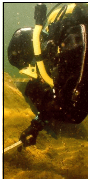
Figure 123. —Diver performing an underwater inspection.
