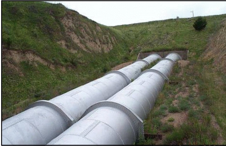
Figure 41. —Penstocks extending through an embankment dam.
