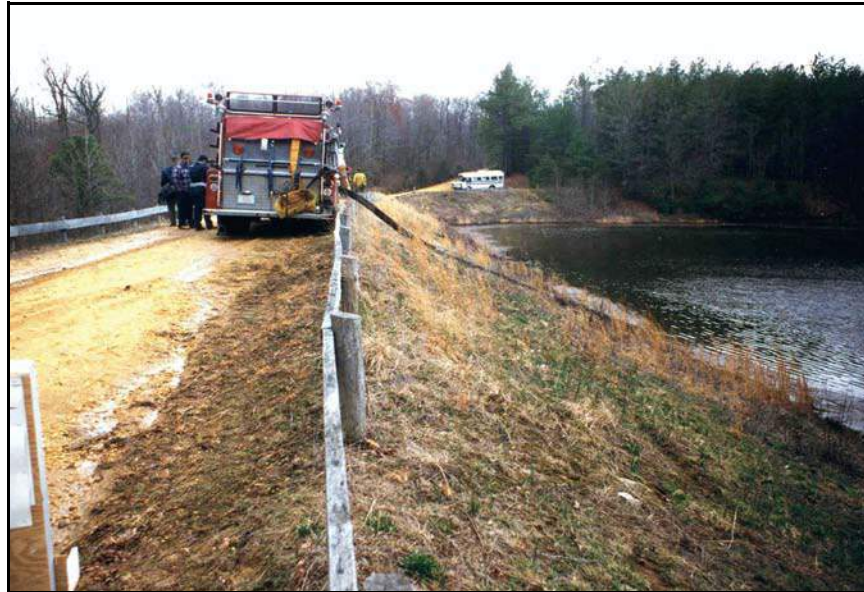
Figure 152. —All available resources may need to be utilized to drain the reservoir in an emergency. Here, the local fire department assists in draining a lake during a thunderstorm after the 45-year old CMP spillway collapsed.
