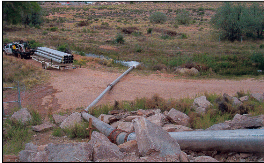
Figure B-61. —Siphon constructed over to crest of the embankment dam for discharging irrigation releases.
