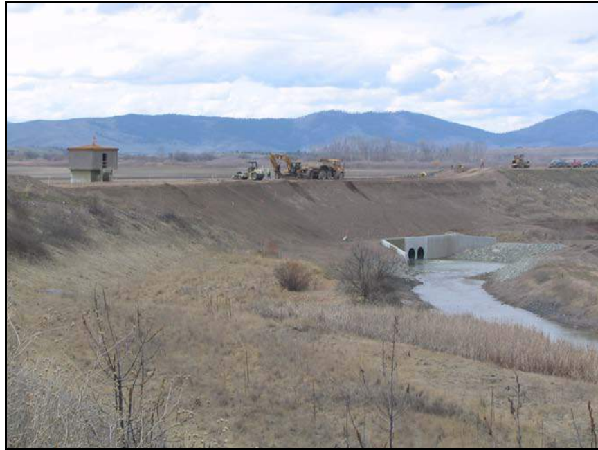
Figure B-58. —Pablo Dam nearing completion.
