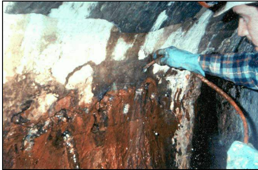
Figure 192. —Injection of urethane grout to stop leakage.
