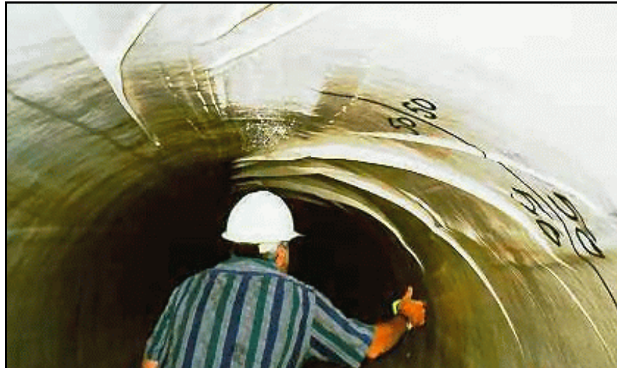
Figure 185. —The calibration hose of this pulled-in-place CIPP developed “fins.” These fins were considered to have an insignificant effect on hydraulic capacity for this particular conduit application and were not removed.
