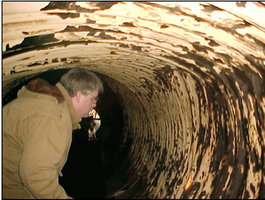
Figure 121. —Inspection of a CMP conduit looking for signs of deterioration.
