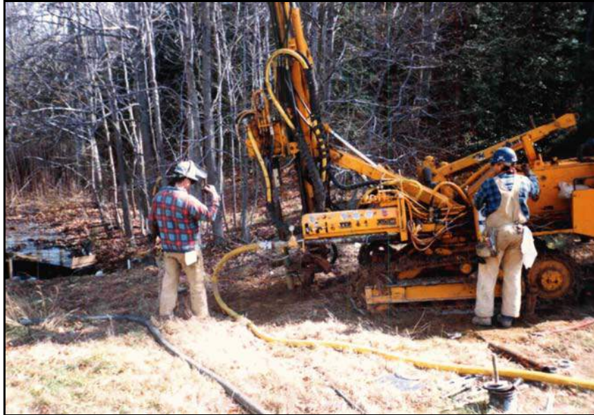
Figure 197. —Abandonment of a conduit by injection of cement grout through holes drilled from the surface of the embankment dam to depths of up to 60 feet.
