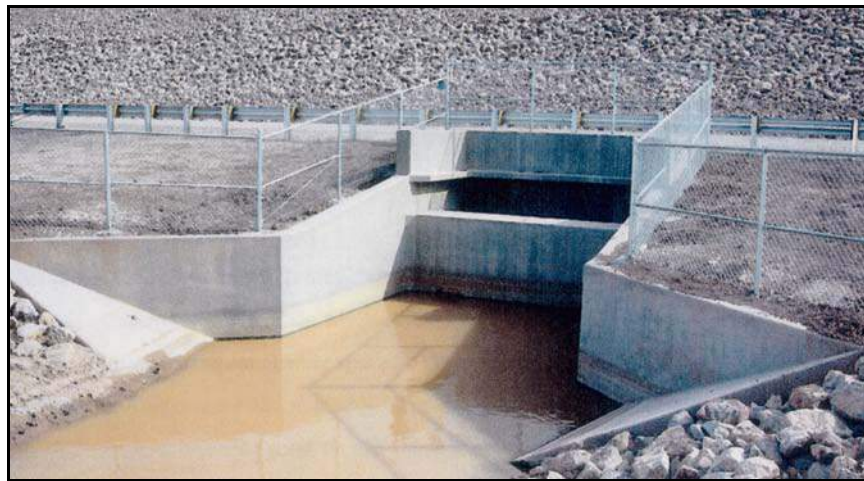
Figure 43. —Typical outlet works terminal structure.
