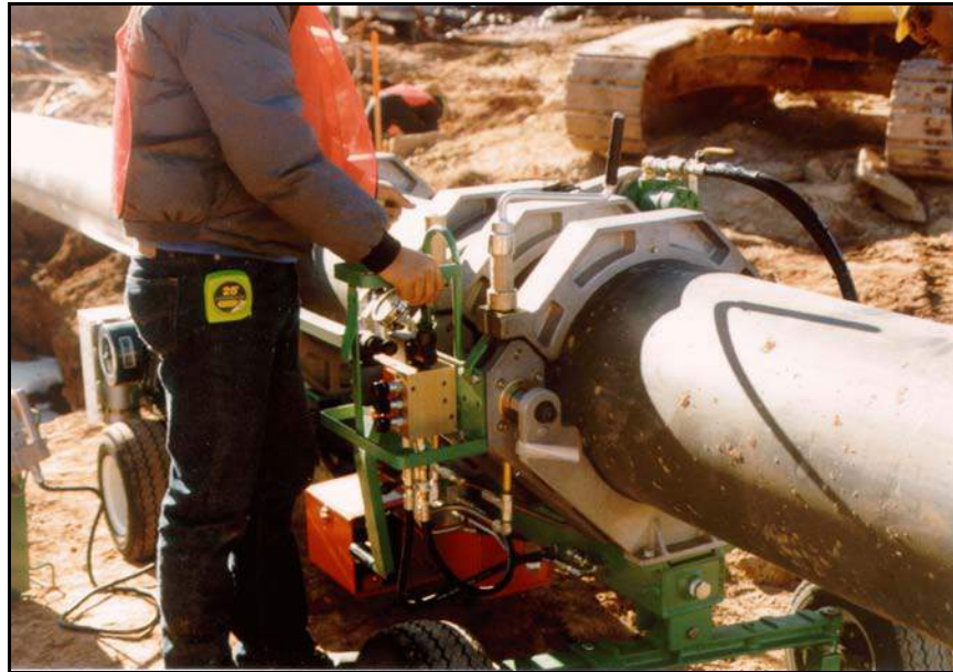
Figure 163. —HDPE pipe joint being fusion welded.
