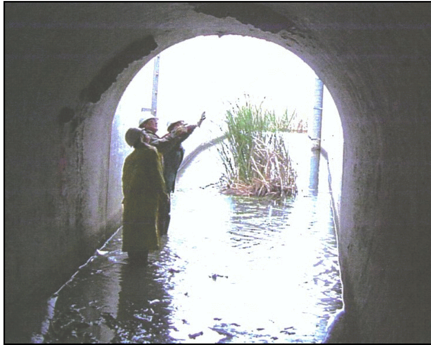
Figure 56. —An example of the interior of conduit shape C.
