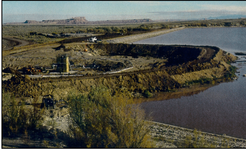
Figure 187. —Cofferdam constructed around the construction area for a new outlet works.
