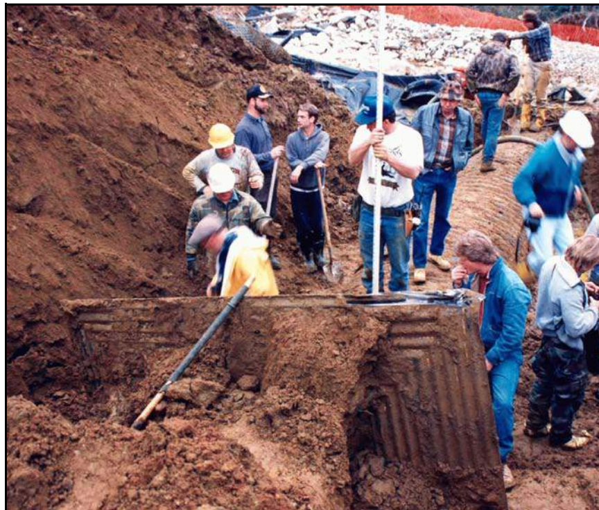
Figure B-8. —Starting at the downstream end of the conduit, two large excavators removed the majority of the earthfill under the watchful eyes of State and local officials, geotechnical engineers, surveyors, lawyers and the pipe manufacture.
