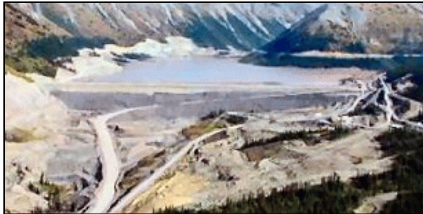
Figure 12. —An example of a tailings dam.
