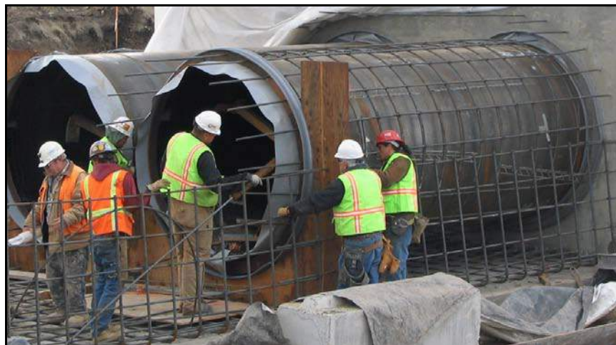
Figure 53. —A multibarrel outlet works conduit under construction.
