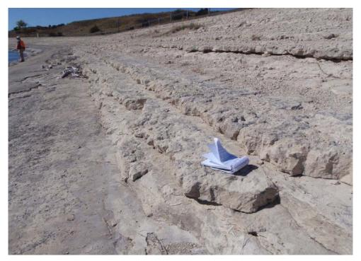
Figure 17.2.2-5. Typical condition of upstream slope protection at Merritt Dam, Nebraska.
