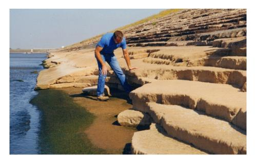
Figure 17.2.2-2. Damaged soil-cement slope protection on the upstream slope at Cheney Dam, Kansas.
