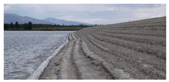
Figure 17.4.2.2.3-1. Soil-cement slope protection at Jackson Lake Dam, Wyoming.
