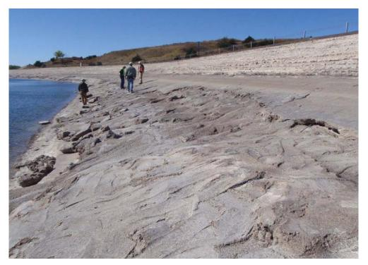
Figure 17.2.2-6. Portion of concrete repairs to soil-cement slope protection at Merritt Dam, Nebraska.
