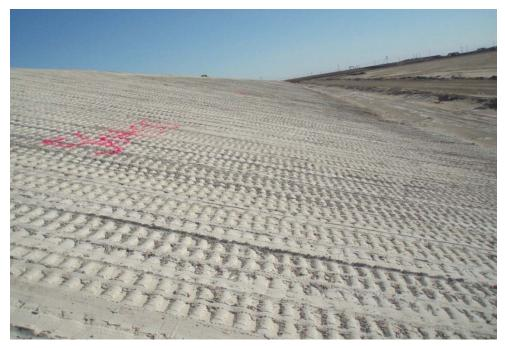
Figure 17.5.3-3 Plating soil-cement at Warren H. Brock Reservoir, California.
