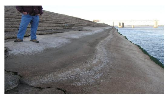
Figure 17.2.2-4. Closeup view of concrete patch on soil-cement slope protection at Cheney Dam, Kansas.
