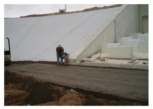
Figure 17.5.6.3-1. Special compaction of soil-cement adjacent to concrete structure at Warren H. Brock Reservoir, California.
