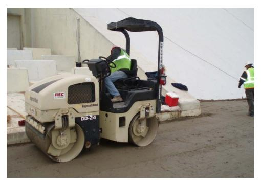
Figure 17.6.3-3. Vibratory steel drum roller used to compact soil-cement at Warren H. Brock Reservoir, California.
