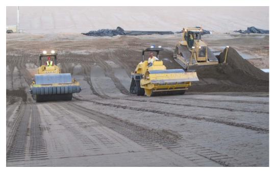
Figure 17.6.3-1. Plating soil-cement placement at Warren H. Brock Reservoir, California.
