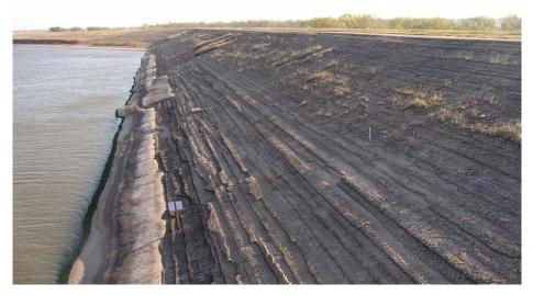
Figure 17.2.2-3. Upstream slope showing soil-cement slope protection and concrete repairs at Cheney Dam, Kansas.
