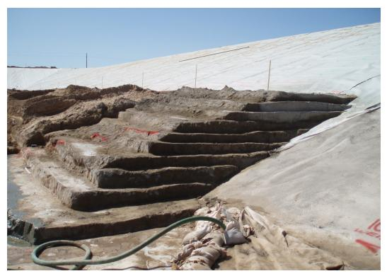
Figure 17.5.5-1. Stairstep soil-cement placement at Warren H. Brock Reservoir, California.
