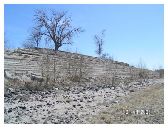
Figure 17.2.2-1. Soil-cement test section at Bonny Reservoir, Colorado.
