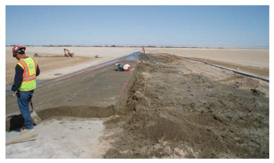
Figure 17.5.5-2. Plating soil-cement placement at Warren H. Brock Reservoir, California. (Note the vertical construction joint.)
