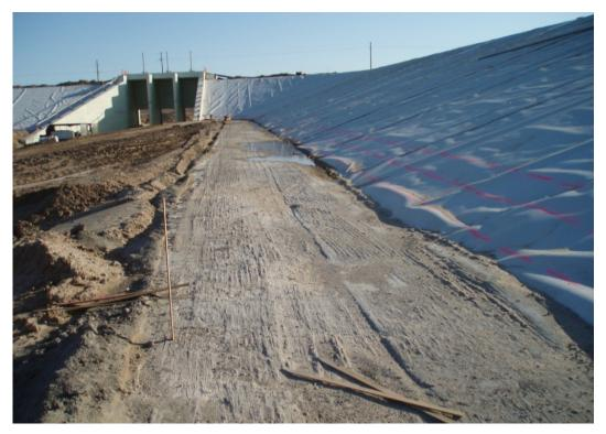
Figure 17.5.7-2. Scarified soil-cement lift at Warren H. Brock Reservoir, California.
