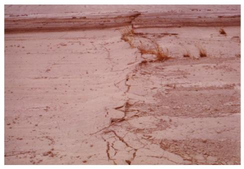
Figure 17.5.5-3. Damaged soil-cement slope protection on the 10H:1V beaching slope at Merritt Dam, Nebraska.
