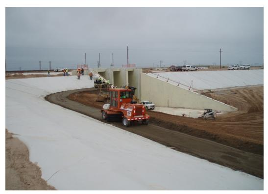
Figure 17.5.7-3. Cleaning soil-cement lift at Warren H. Brock Reservoir, California.
