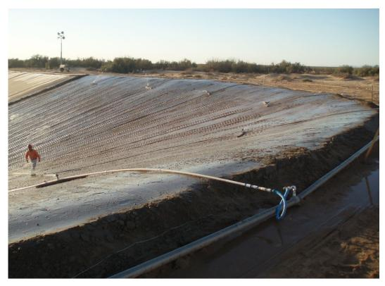
Figure 17.6.4-1. Sprinklers used for water cure at Warren H. Brock Reservoir, California.
