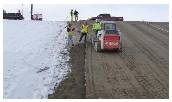
Figure 17.6.5-1. Trimmed vertical construction joint at Warren H. Brock Reservoir, California.
