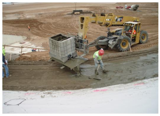
Figure 17.5.7-1. Spreading of cement slurry bonding agent at Warren H. Brock Reservoir, California.
