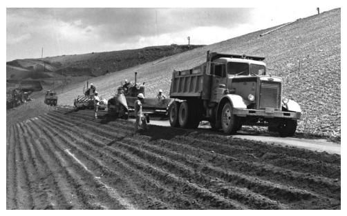
Figure 17.6.3-2. Placement of soil-cement slope protection, Starvation Dam, Utah.
