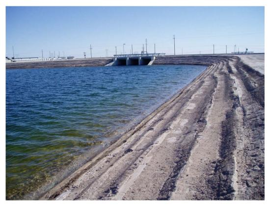
Figure 17.5.3-2. Stairstep soil-cement at Warren H. Brock Reservoir, California.
