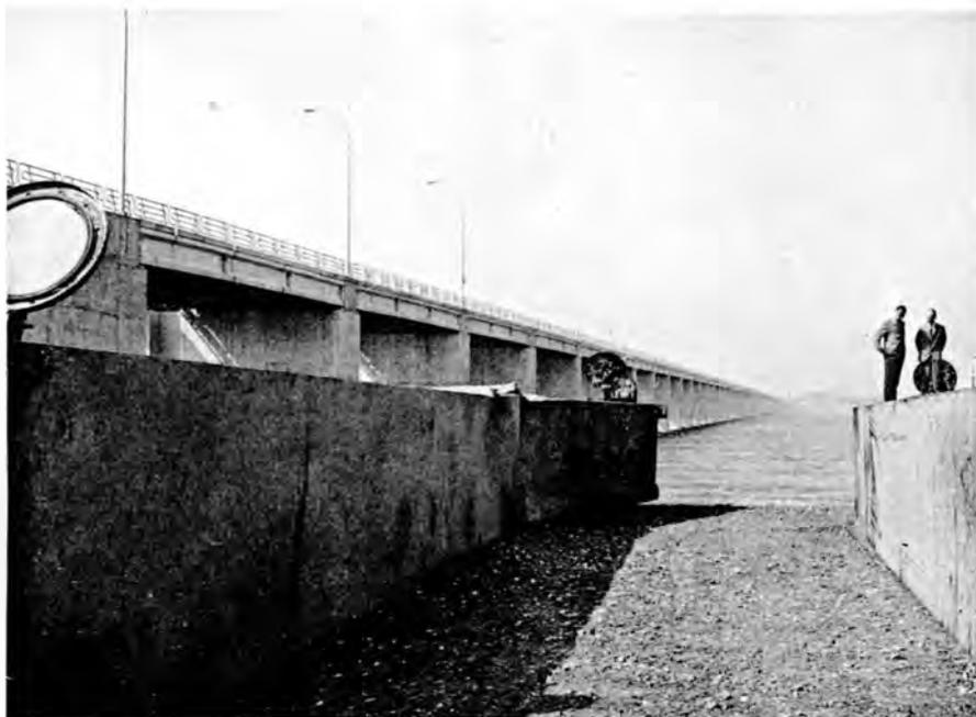
Figure 17. Steel stop-log, 88 ft long, broken by ice impact (1967).
