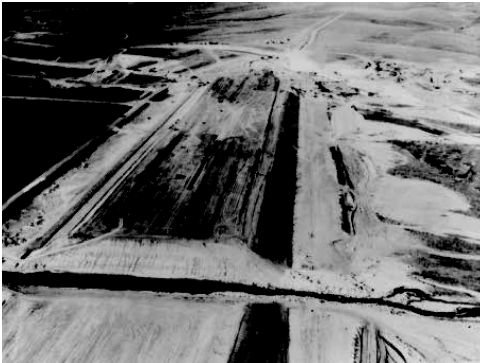
Figure 10.6.7.3-1 Bonny Dam, Colorado. Temporary diversion channel. USBR 1948
