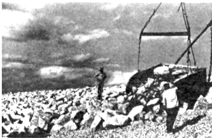
Figure 10.6.8.2.1-1 Dragline with skip placing riprap [1].
