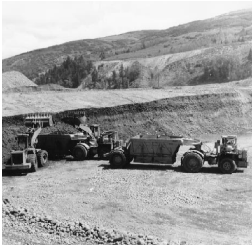
Figure 10.5.1.1.1-3 Jordanelle Dam, Utah. Two model 992C Caterpillar front end loaders loading zone 4 (gravel and cobble fill) from borrow into a model 540 Dart belly dump truck. This type of loading operation, with steep face of the borrow area, can be used to get a well-mixed fill from a layered deposit. August 1990
