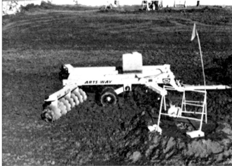
Figure 10.6.1.3.3-1 New Waddell Dam, Arizona. Disk plow used for conditioning and scarifying impervious fill.
