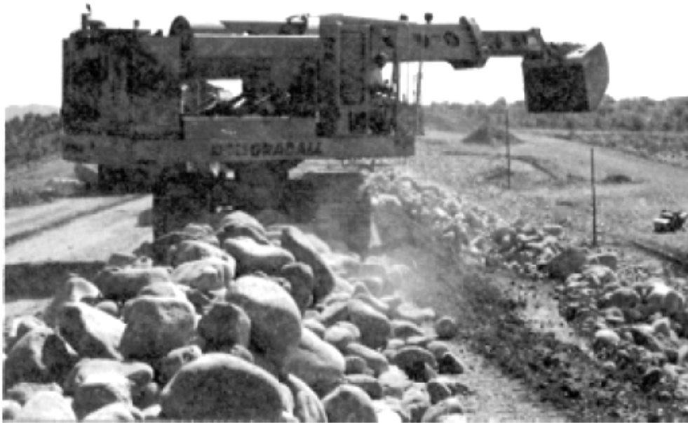
Figure 10.6.8.2.1-3 New Waddell Dam, Arizona. Gradall used to place slope protection. USBR 1992
