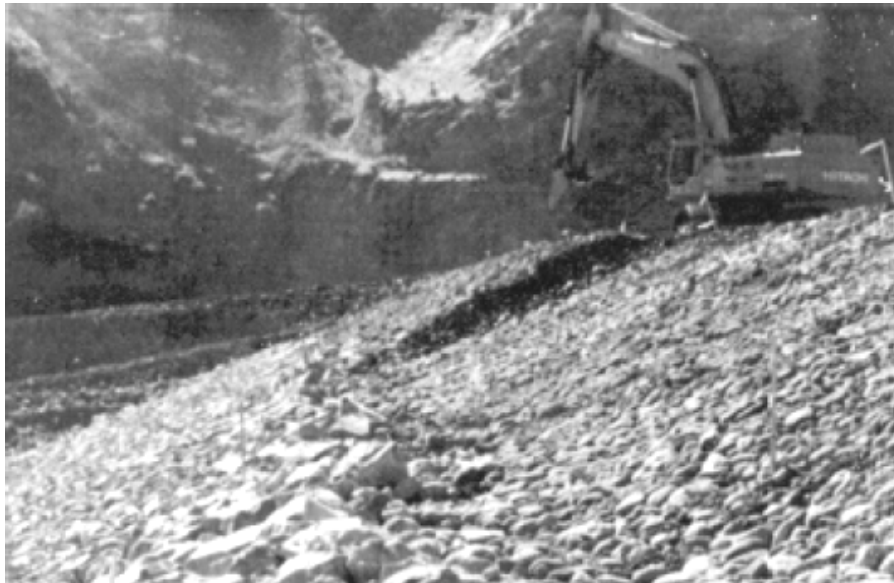
a. Shaping of embankment surface in preparation for placing riprap.
