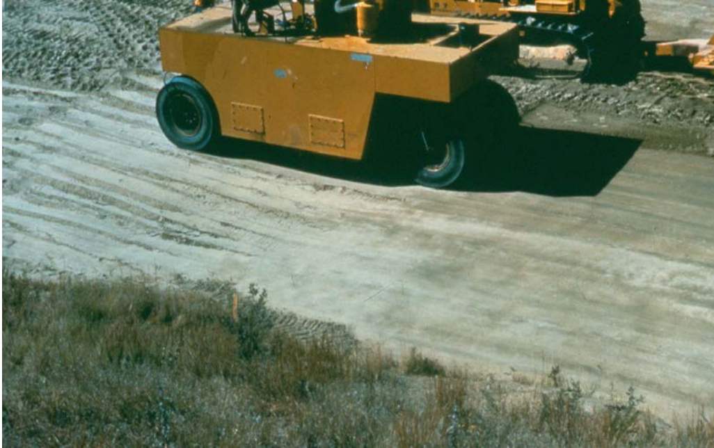
Figure 10.6.1.1-3 Pneumatic (rubber-tired) roller. Pneumatic tired rollers are sometimes used on impervious fill with scarification of the top surface of the lift after the lift is compacted.
