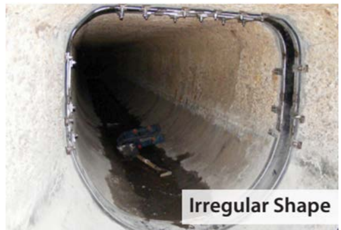
Figure 6. Example of a Non-Circular Mechanical Rubber Seal (photo courtesy of HydraTech).
