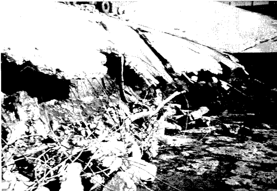
b. Closeup view of spillway damage
