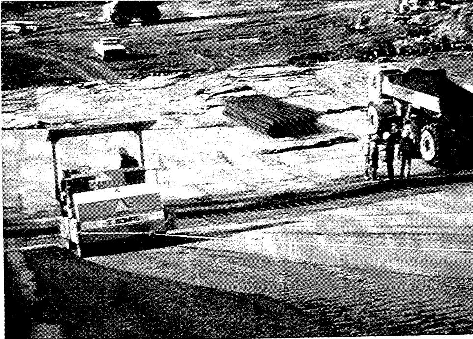
Figure 4. RCC compaction on the downstream slope, Toutle River Dam
