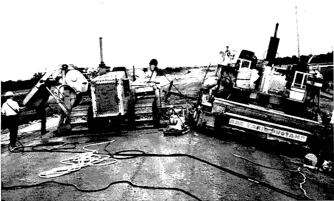
Figure 15. RCC paver connected to a bulldozer for paving slopes at Barker Dam
