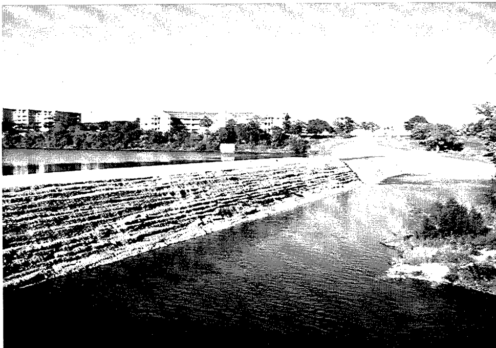
Figure 11. Condition of the RCC following overtopping, Kerrville Ponding Dam
