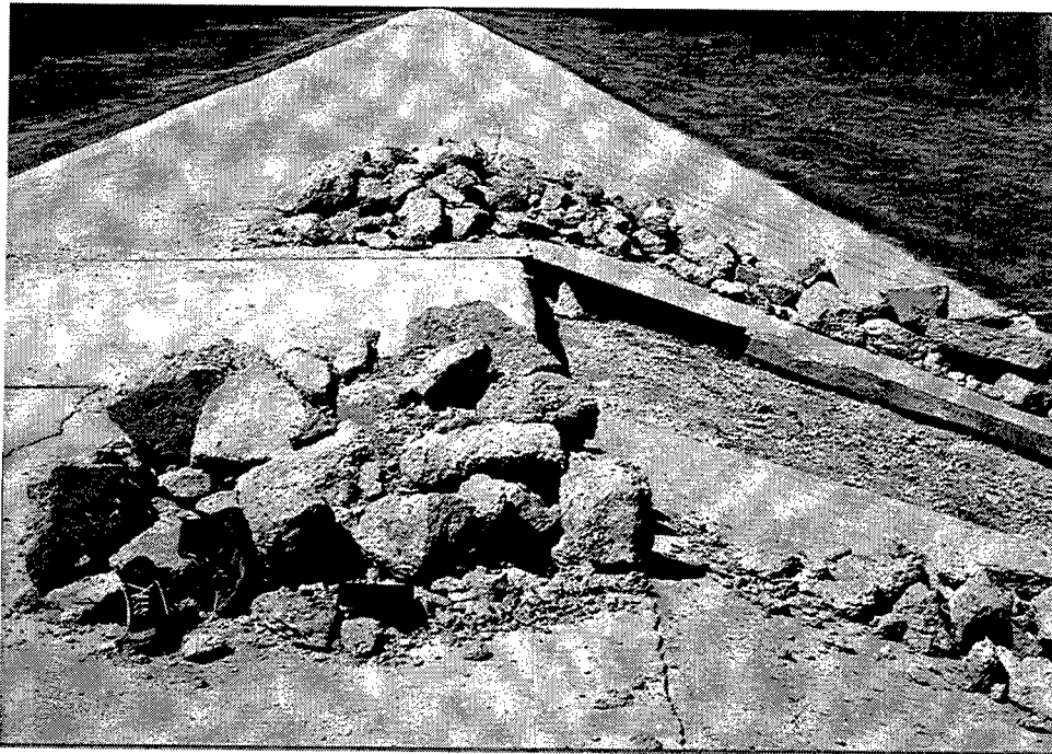
Figure 20. Removal of spalled RCC and replacement with new concrete, Barker Dam
