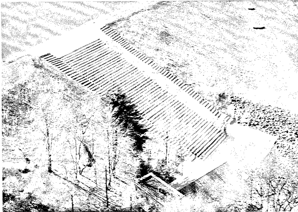
Figure 53. Completed spillway, Ringtown No. 5 Dam
