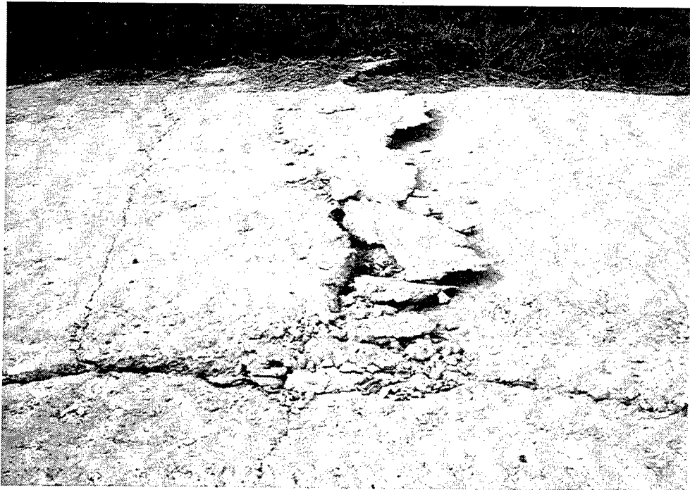
Figure 17. Buckling blowups in RCC at Addicks Dam
