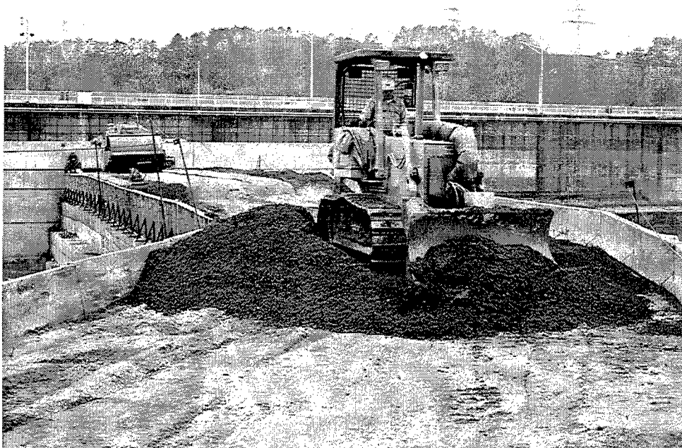
Figure 45. Spreading and compaction of RCC at Nickajack Dam
