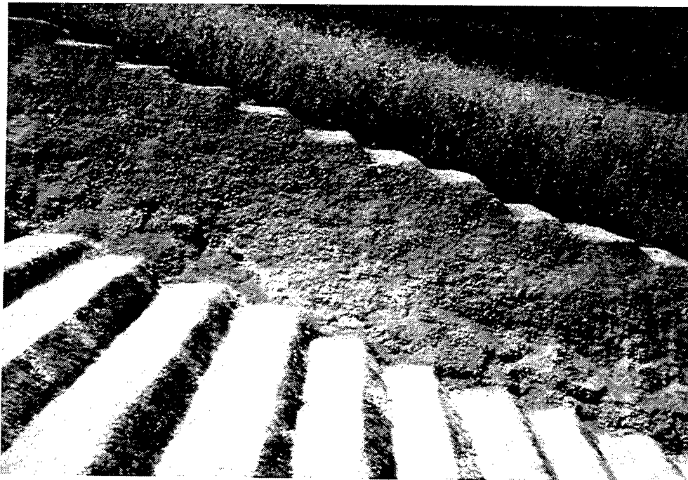
Figure 52. Completed steps and wall, Ringtown No. 5 Dam
