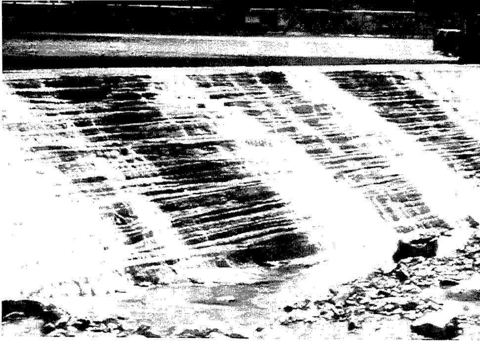
Figure 2. Downstream face of Ocoee Dam with RCC overtopping protection
