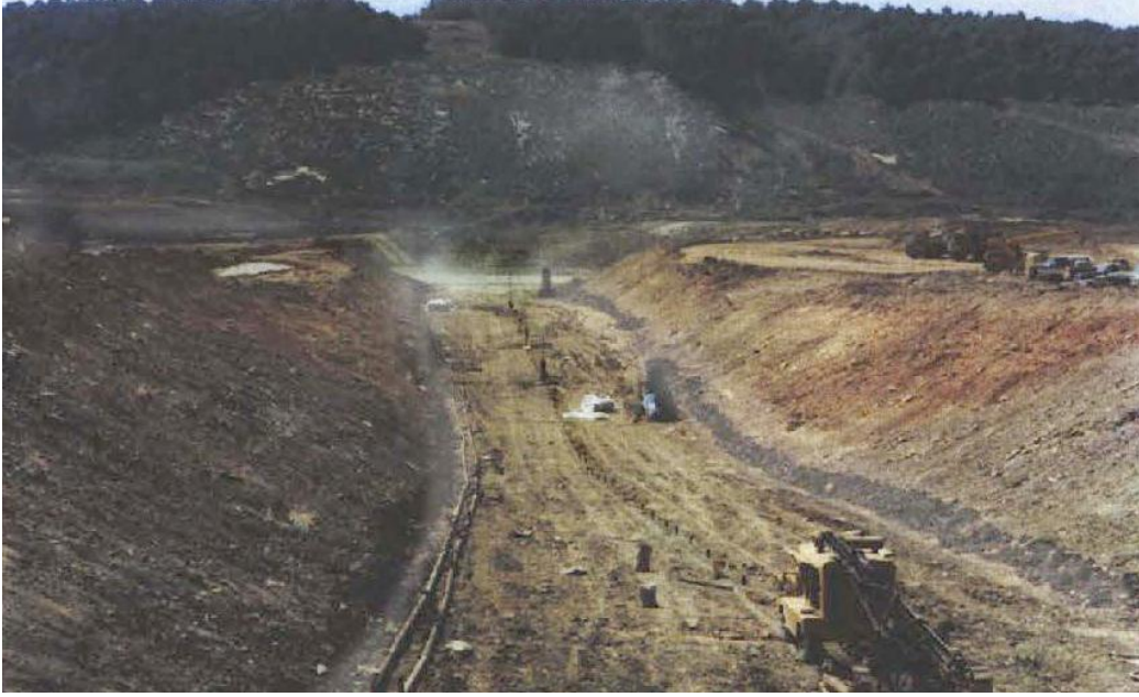
Figure A-4 – Photograph of curtain grouting at McGee Creek Dam
