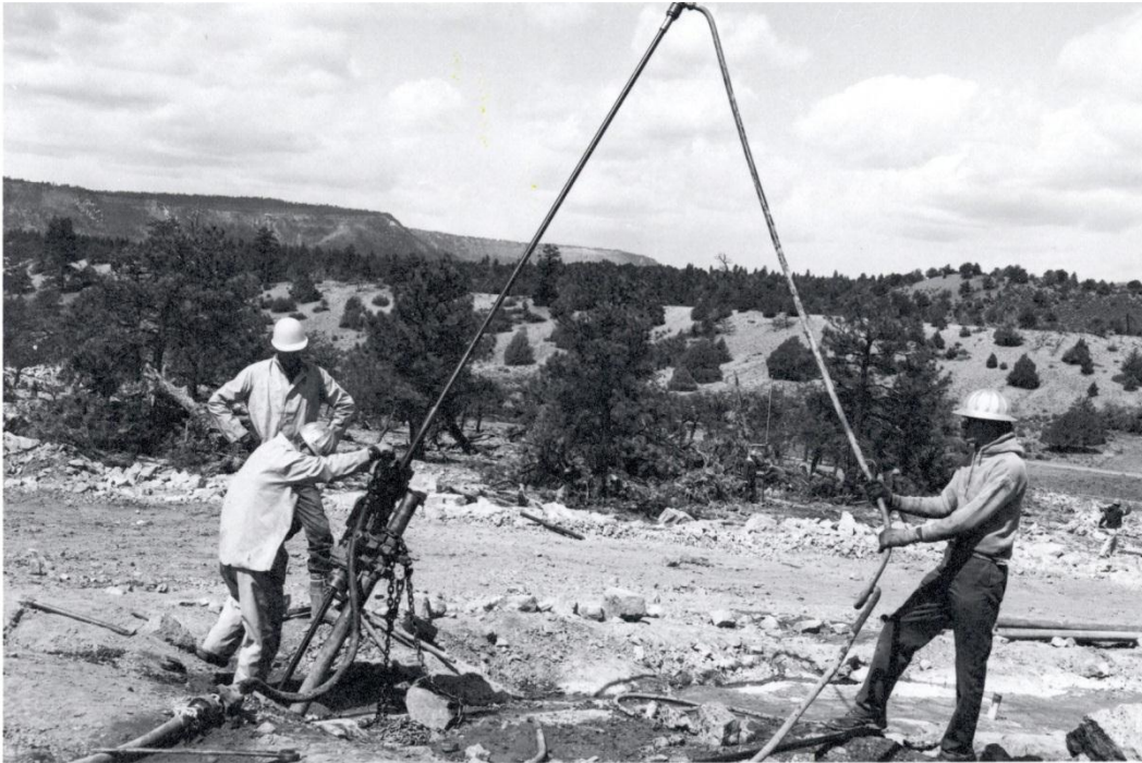
Figure A-9 – Photograph of grout hole construction at Heron Dam
