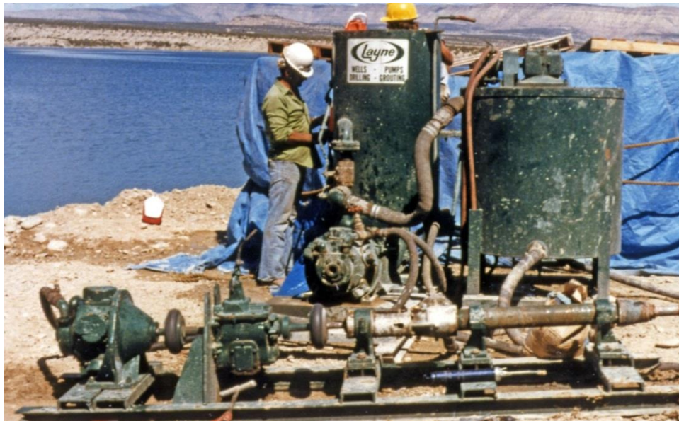
Figure 15.12-1. Portable batch plant at Starvation Dam.
