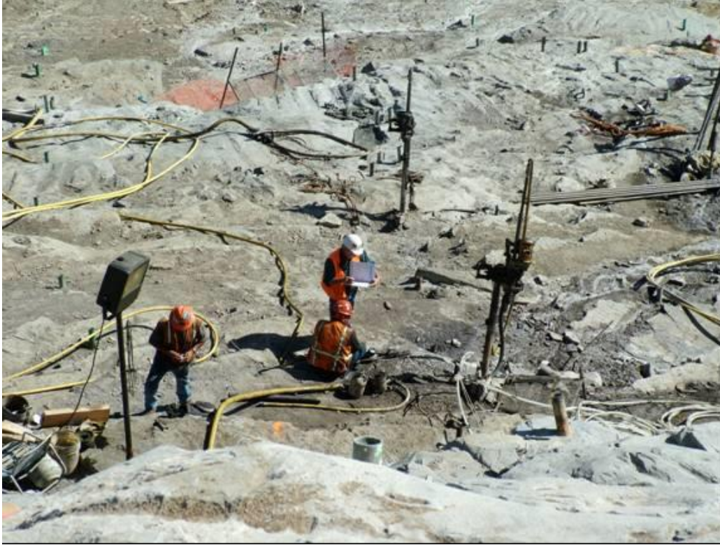
Figure 15.7.6.1-2. Drilling and grouting of blanket grout holes on a Reclamation project.
