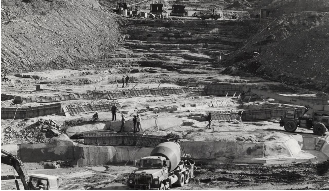
Figure A-1 – Photograph of core trench construction at Ridgway Dam.
