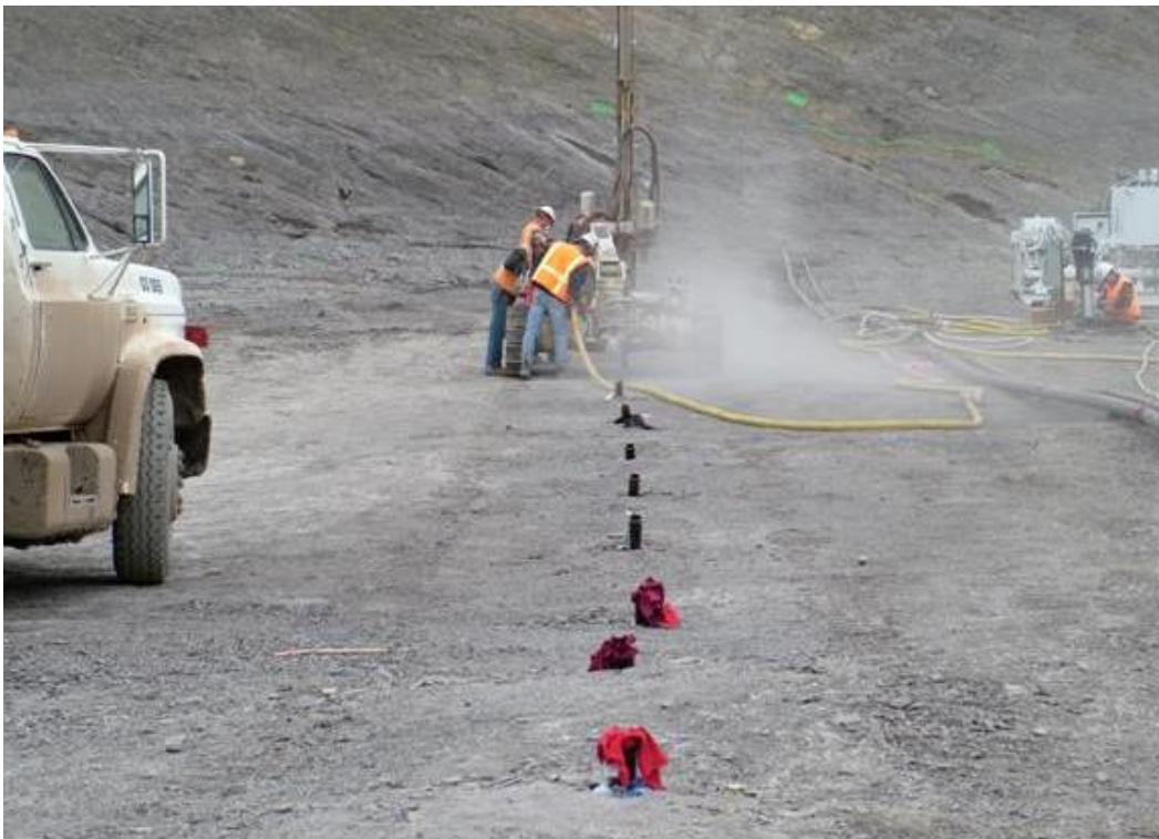
Figure 15.6.8-2. Contractor setting standpipes along a single row grout curtain.
