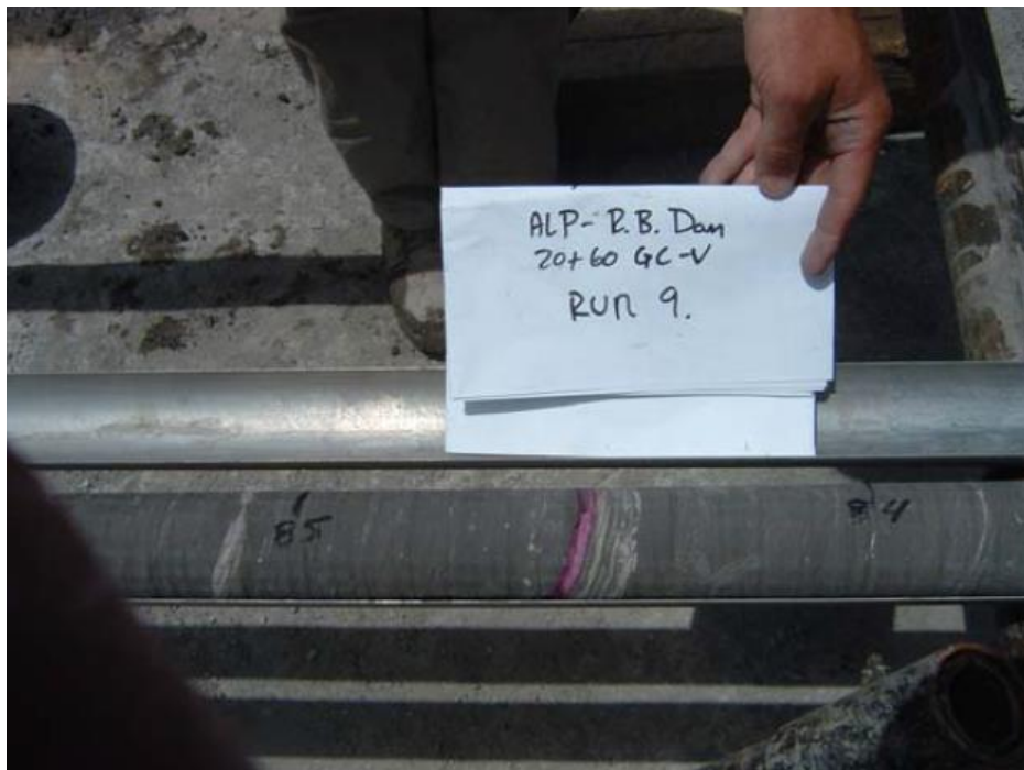
Figure 15.5-1. Photo illustrates grout infilling (shown in purple) of joint within a grout check hole
