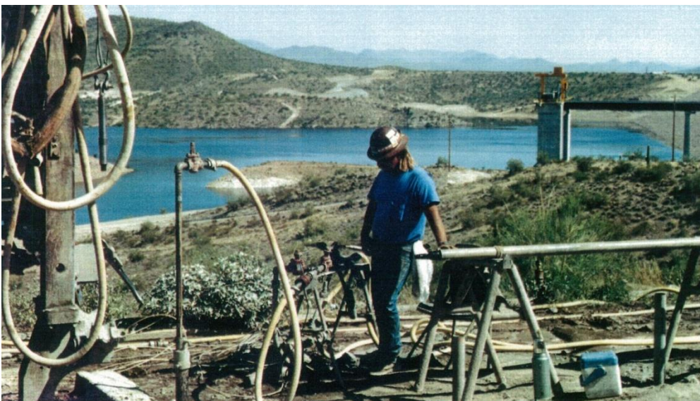
Figure A-14 – Photograph of grouting performed along right abutment ridge
