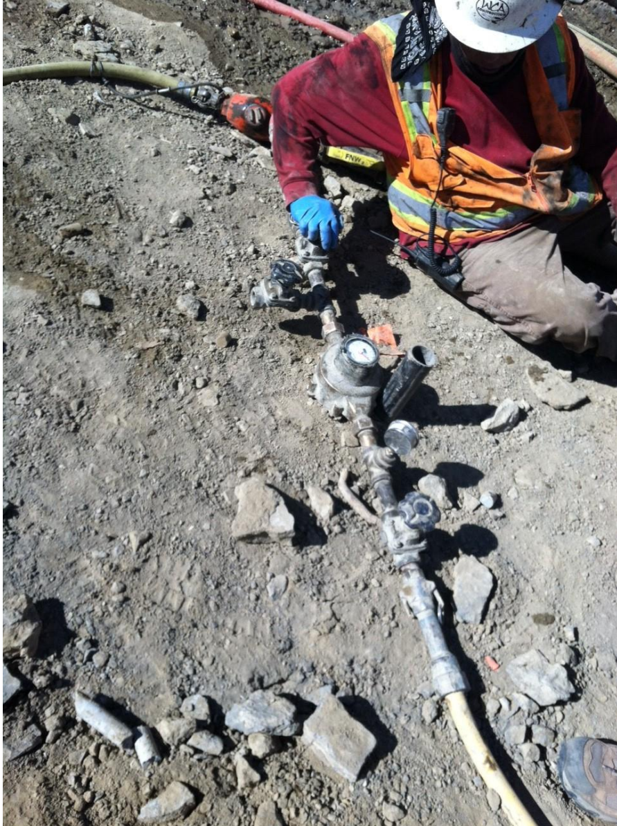
Figure 15.6.7.2-1. Typical manifold configuration used by contractors for water tests.
