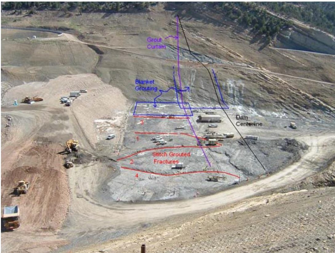
Figure 15.1.2-1. Overview of grouting operations at Ridges Basin Dam.
