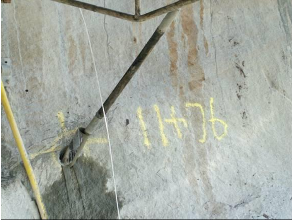
Figure 15.12.10-1. Inflatable packer being placed into grout hole.
