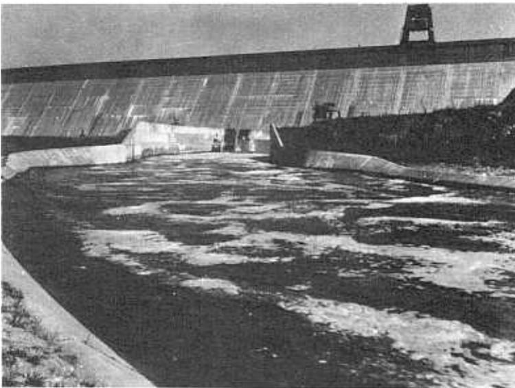
$Q=3,900$  c.f.s.—after wave suppressor was installed.
