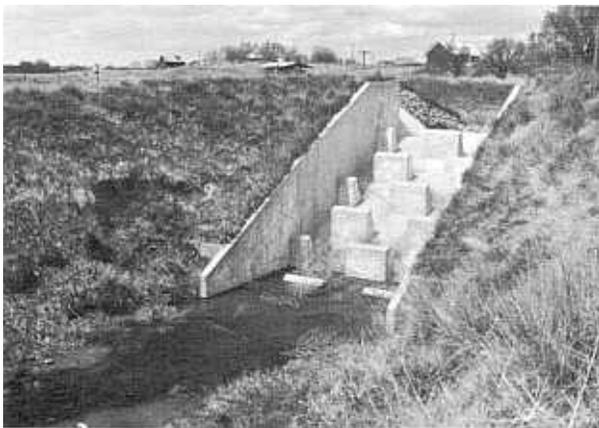
Structure after 4 years of operation. Performance has been satisfactory. Design discharge 625 c.f.s. Bostwick Franklin Canal, Drain F-10.1, Sta. 84+88.
