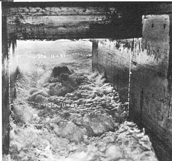
FIGURE 92.—Boysen Dam: left valve of outlet works basin discharging 732 c.f.s.—looking downstream.
