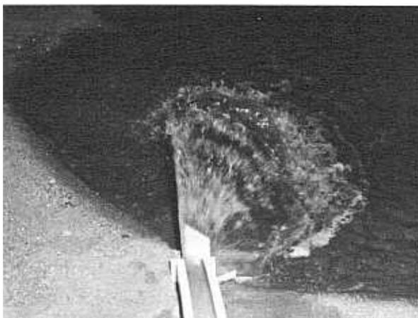
FIGURE 143. *Dispersion-type flip bucket— $Q=24,000$  c.f.s.*
