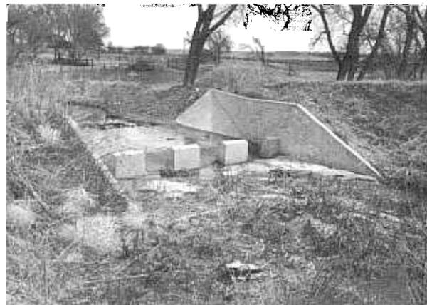
Structure after 5 years of operation. Performance has been satisfactory. Design discharge 1,100 c.f.s. Bostwick Franklin Canal, Drain F-14.9, Sta. 5+20.
