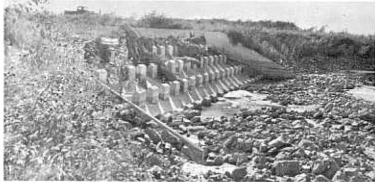
Erosion after a year of operation has exposed one more row of blocks. Rocks were sorted from finer material which moved. Rubbish has collected by September 1957.
