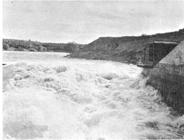
90-inch left valve 100% open, discharging 2,300 c.f.s., approx. Reservoir elevation 301.83. Tail water elevation 183.0.
