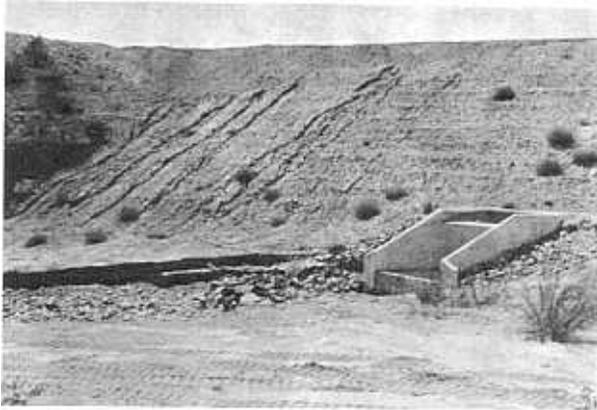
FIGURE 168.—Impact-type stilling basin structure, Picacho North Dam, following flood of August 20, 1954.
