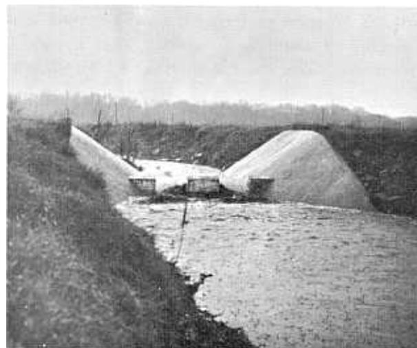
Performance of structure during rainstorm. Discharge 81 c.f.s. in May 1959. Design discharge 400 c.f.s.
