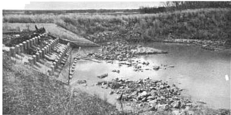
Erosion did not continue at original rate, and is no more severe after 2½ years of operation in April 1959.
