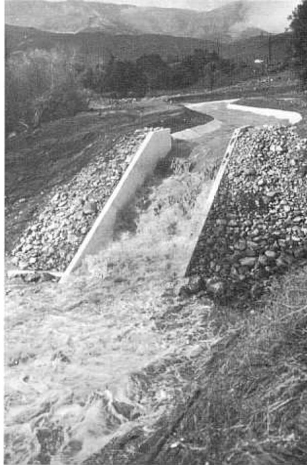
▶ Robles-Casitas Canal between Sta. 294 and Sta. 298 with 500 c.f.s. discharging into Santa Ana Creek. Waves in canal section occasionally splash over top of canal concrete lining.
