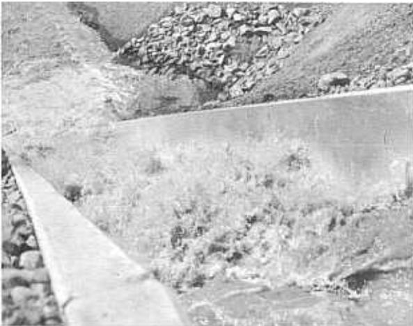
Baffled chute at Sta. 667+78, Extension Boulder Creek Supply Canal, Colorado-Big Thompson project, designed for 200 c.f.s. Discharges of 150 c.f.s. (upper left) and 100 c.f.s. (lower left) show excellent performance in both instances.
