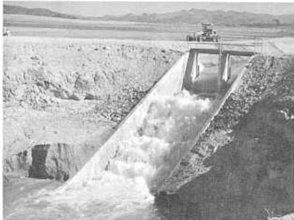
FIGURE 126.—Construction and performance of baffled chutes.
