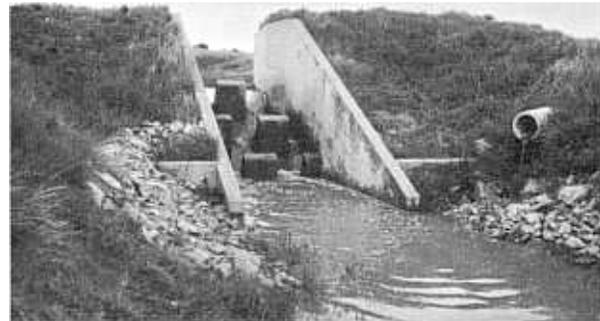
Discharge about 3 c.f.s. Reports received indicate that structure performs well for large discharges.
