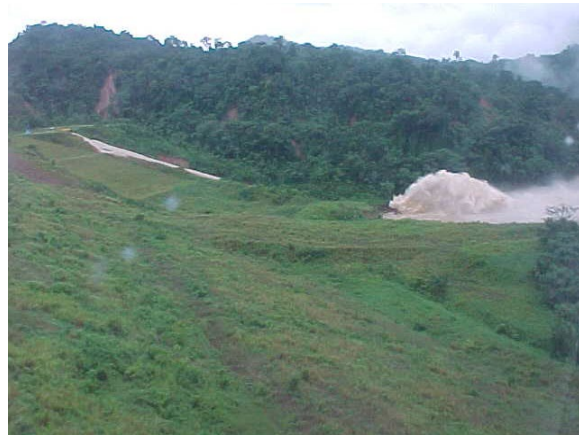
1999 Stilling Basin Sweepout (erosion in downstream channel creating “roster-tail”). Dam Failed due to Flood-induced Chute Wall Overtopping – El Guapo Dam, Venezuela (courtesy of Ing. Alejandro Hitcher).
