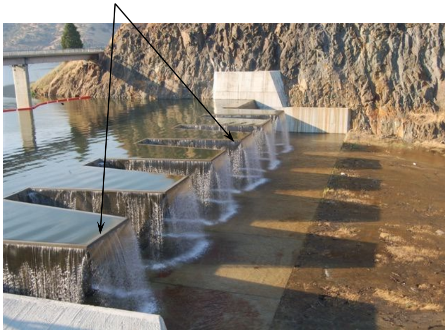
Fusegate spillway, Terminus Dam, California (courtesy of the U.S. Army Corps of Engineers, Sacramento District, Rick Poepelman).
