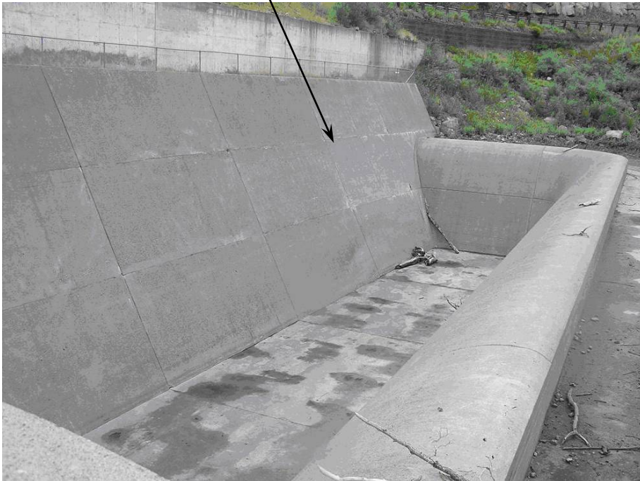
Side-channel service spillway, Paonia Dam, Colorado
