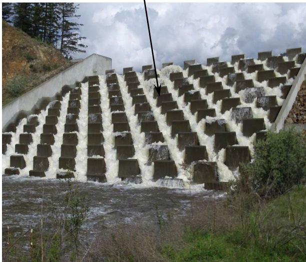
Baffled apron service spillway, Conconully Dam, Washington
