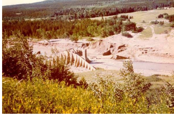
1964 Dam Remnant after Flood-induced Overtopping Failure – Lower Two Medicine Dam, Montana.
