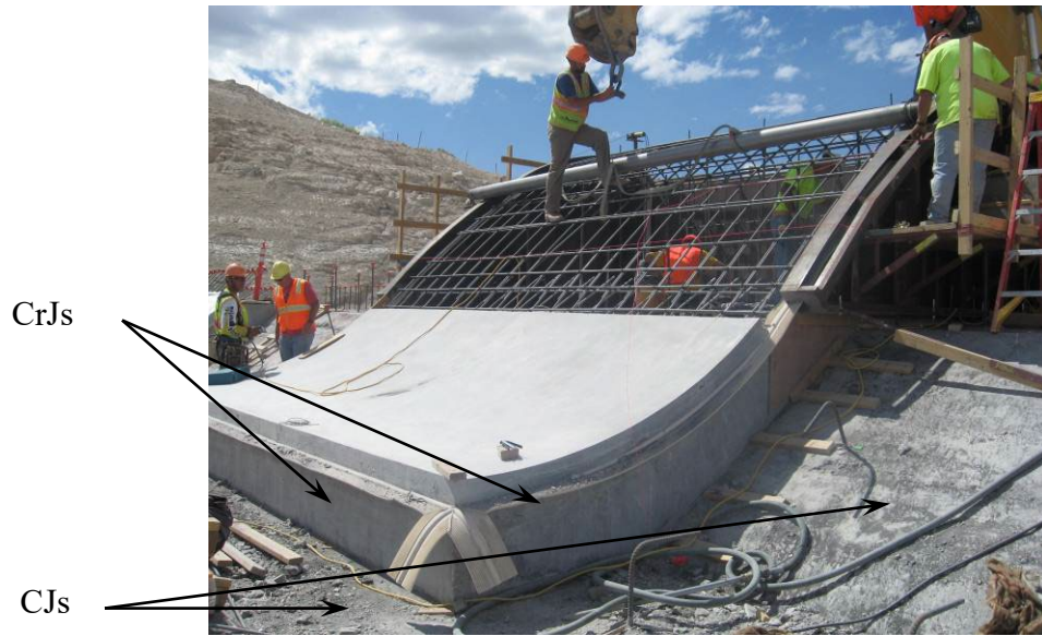
Glendo Dam, Wyoming: construction of new auxiliary spillway
