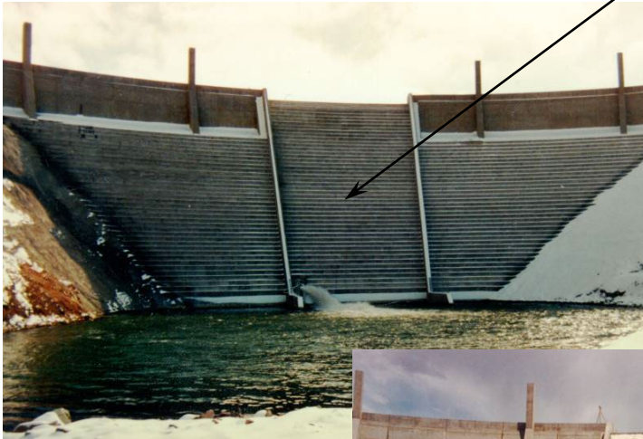
Stepped service spillway integral with concrete dam, Santa Cruz Dam (New Mexico Stream Commission), New Mexico
