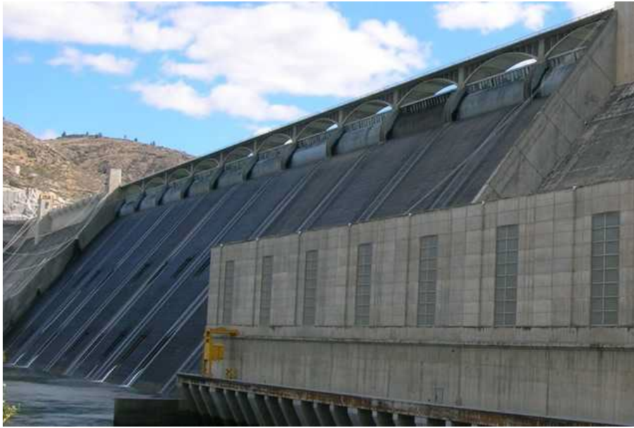
Grand Coulee Dam, Washington: drum gated service spillway
