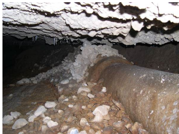
Loss of Foundation beneath Spillway Chute due to Internal Erosion – Reclamation dam.
