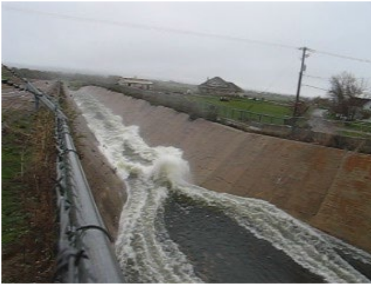
2005 spillway operation. Standing wave at downstream end of transition with cross waves downstream of standing wave – Hyrum Dam, Utah.
