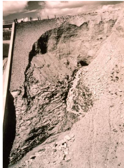
1965 Dam Internal Erosion Incident adjacent to Spillway during Normal Operations – Fontenelle Dam, Wyoming.
