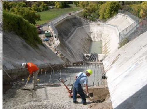
Reclamation Dam – Void below spillway chute floor; ground penetrating radar (GPR) identifying voids; and spillway chute foundation and floor replacement to mitigate foundation piping and high potential of stagnation pressure failure
