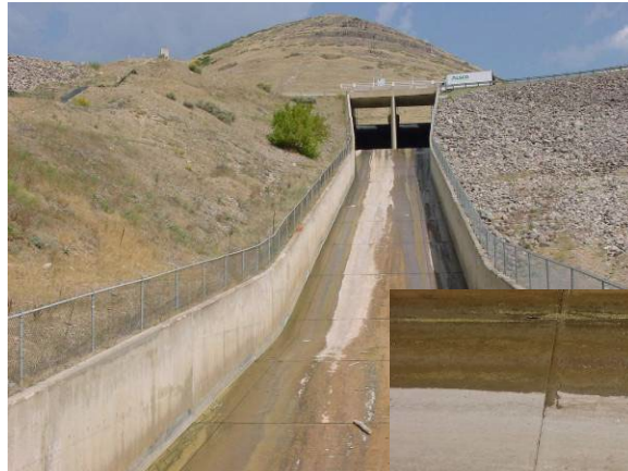
Spillway Chute Damage due to Thermo-expansion/contraction—Deer Creek Dam, Utah
