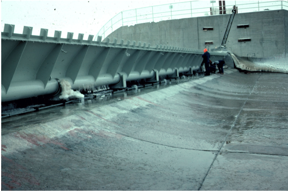
Figure 3.9.1.1-4. Crest gate – bascule type.
