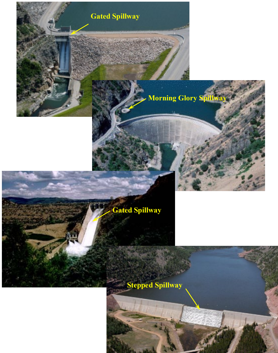
Figure 3.2.1.1-1. Service spillways, from top to bottom: Pineview Dam, Utah; Monticello Dam, California; Echo Dam, Utah; and Upper Stillwater Dam, Utah.
