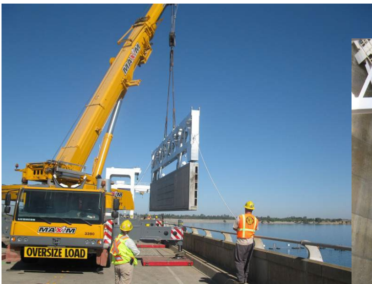
Folsom Dam, California: installation of metal stoplogs
