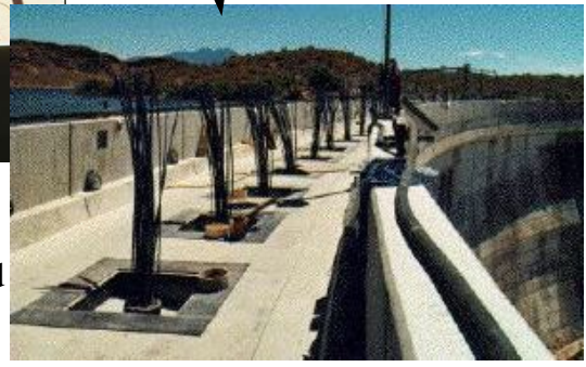
Stewart Mountain Dam Modifications, AZ – 1992 Stabilizing dam and modified existing river outlet works.
