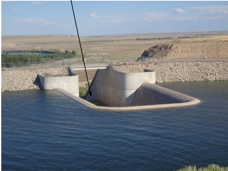
Bathtub service spillway, Fontenelle Dam, Wyoming.
