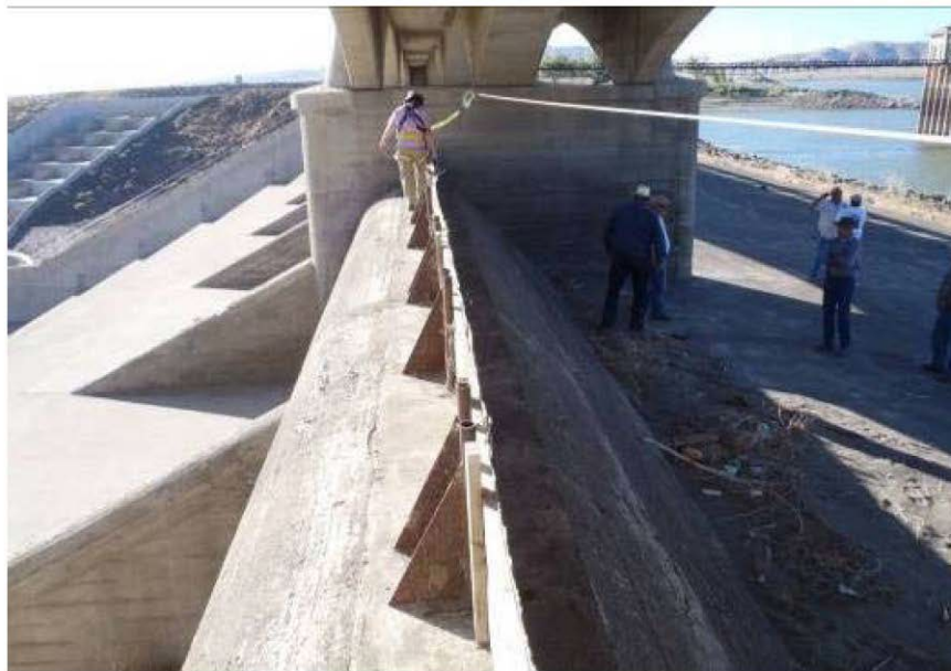
Figure 3.9.1.4-2. Flashboards – Lahontan Dam spillways.
