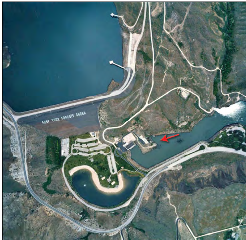
Figure A-43.—Aerial view of Lucky Peak Dam. The arrow denotes the location of the six slide gates and flip buckets.
