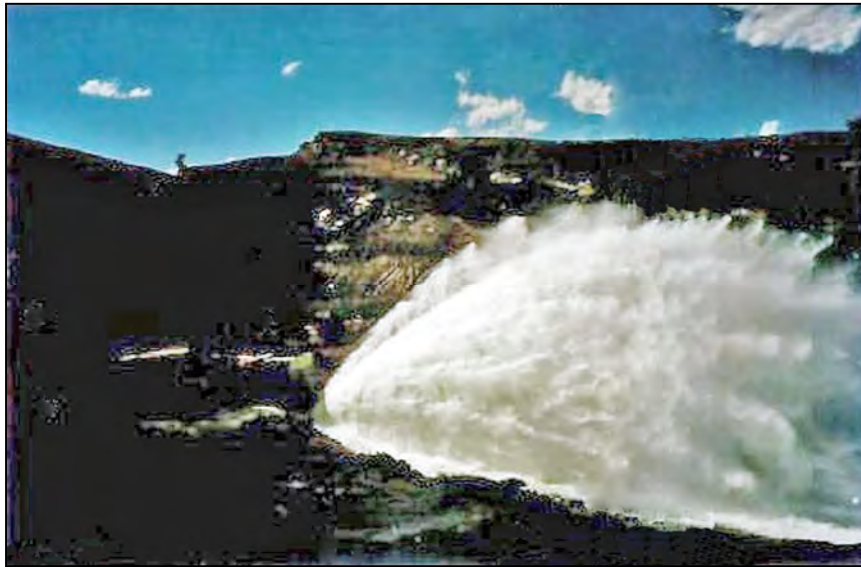
Figure 75.—Fixed-cone valve discharging at a large opening.
