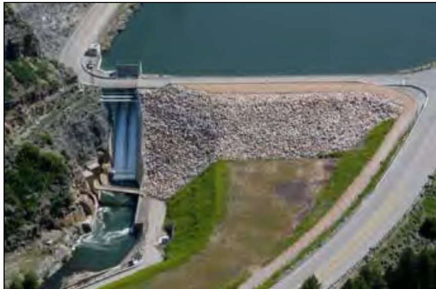
Figure A-75.—Downstream face of Pineview Dam.
