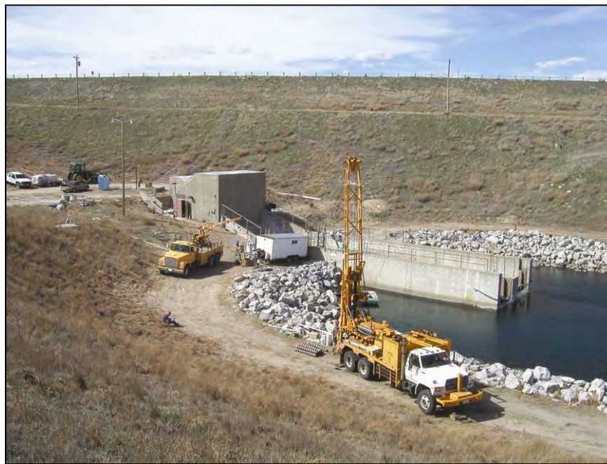
Figure A-124.—River outlet works stilling basin and control house at Virginia Smith Dam.
