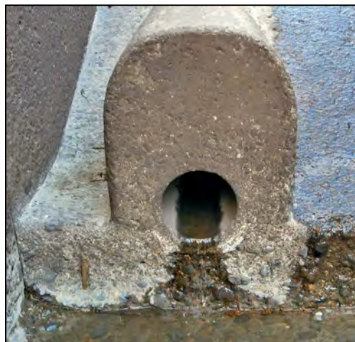
Figure 21.—Looking upstream at a chute block located at the upstream entrance of a stilling basin. A structural underdrain exits from the downstream face of the chute block.
