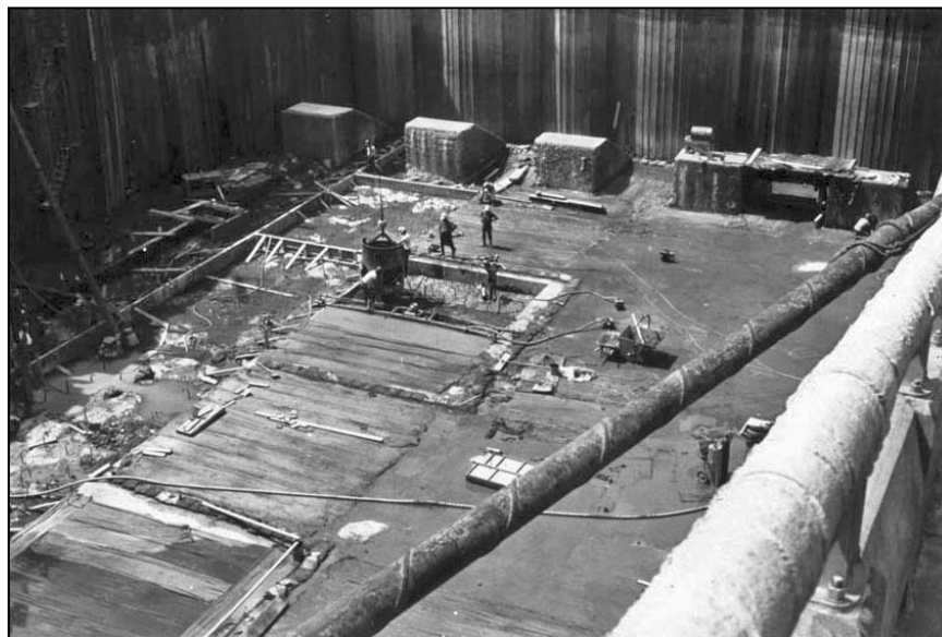
Figure A-40.—General view of repair operations.
