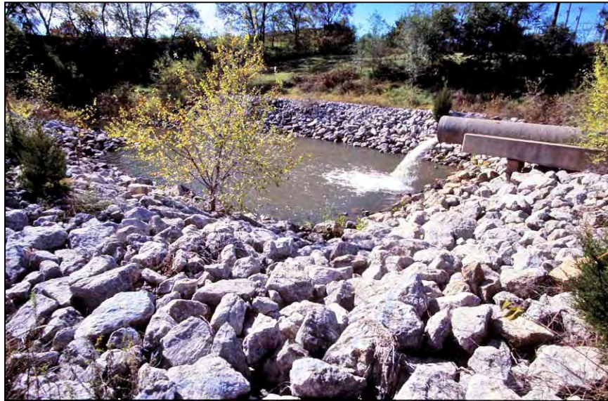
Figure 59.—A riprap-lined plunge basin.
