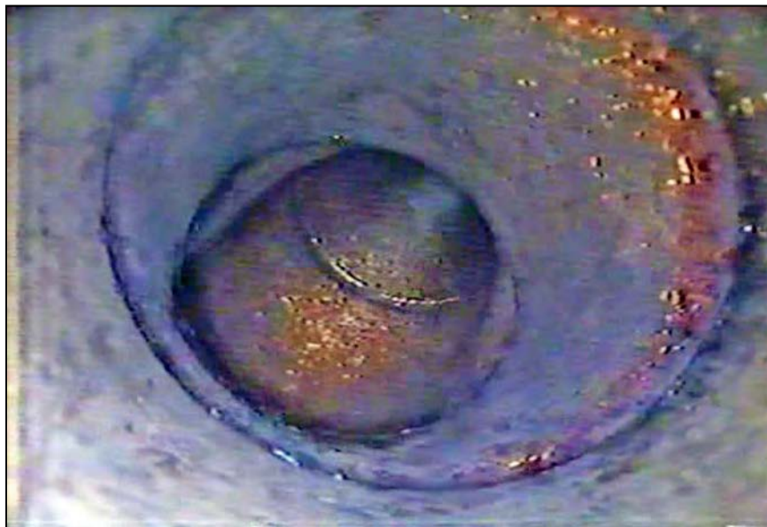
Figure A-109.—View looking vertically downward at the second bend inside Underdrain No. 1 (rightmost drain) in the outlet works stilling basin.
