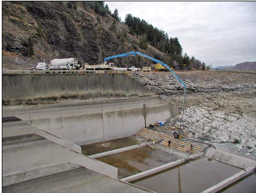
Figure A-71.—Concrete being pumped to forms for repairs to dentate sill.
