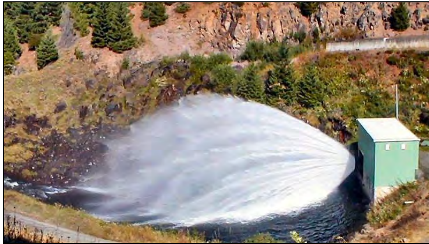
Figure 11.—Flow emerging from a Howell-Bunger valve.
