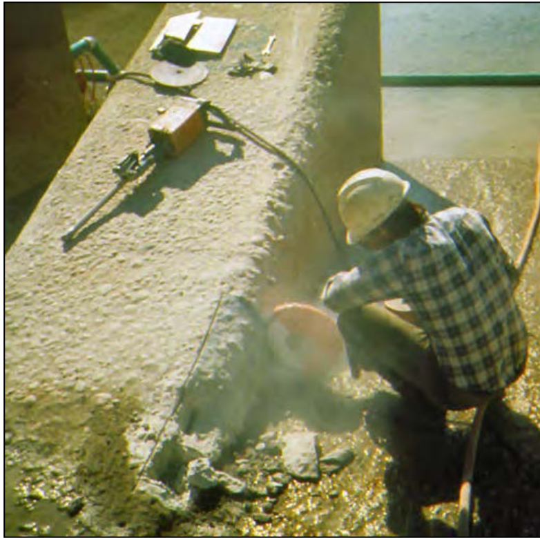
Figure 171.—Sawcutting the perimeter of spalled concrete prior to removal of concrete.
