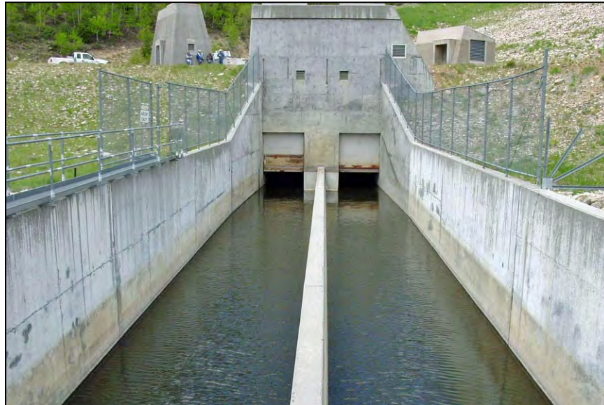
Figure 25.—Splitter wall separating discharge from two conduits.
