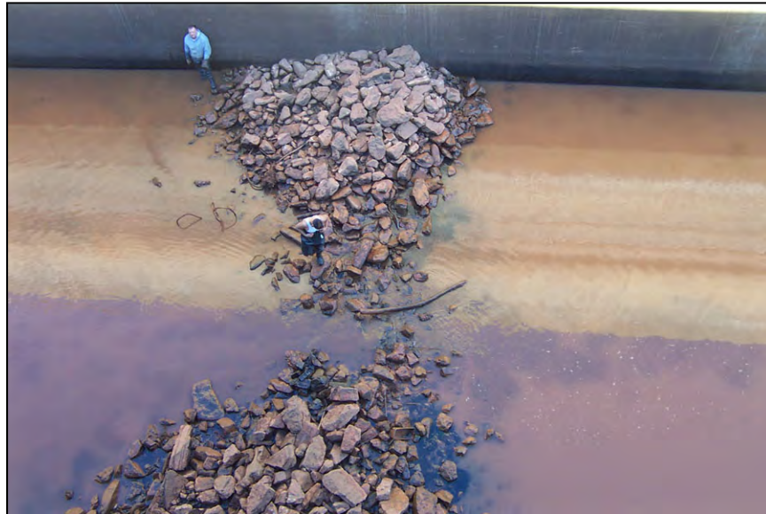
Figure A-61.—Most of the rocks and gravel were located on the downstream two-thirds of the basin floor.
