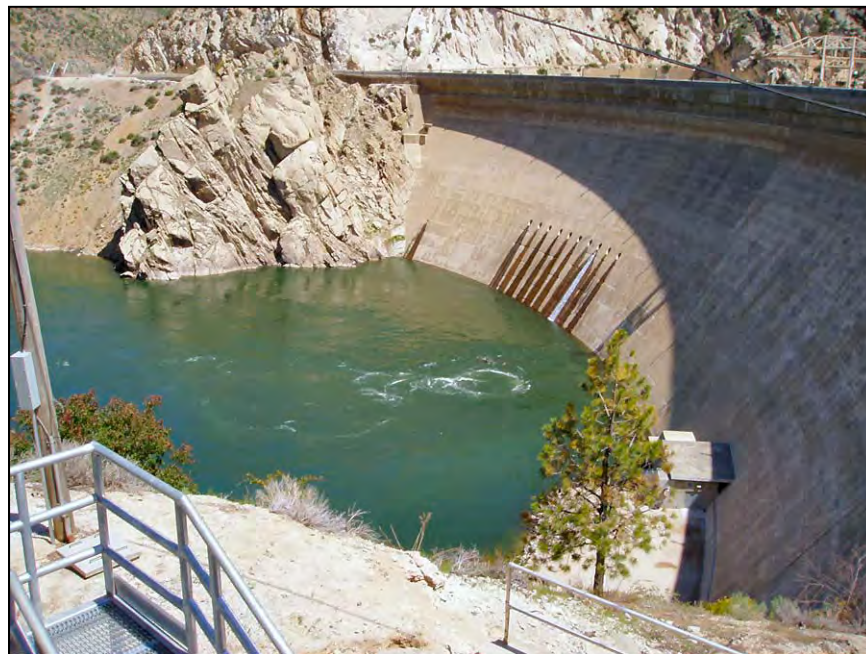
Figure 111.—Clamshell gates operating under 50 feet of submergence. No air was entrained during submerged discharge.
