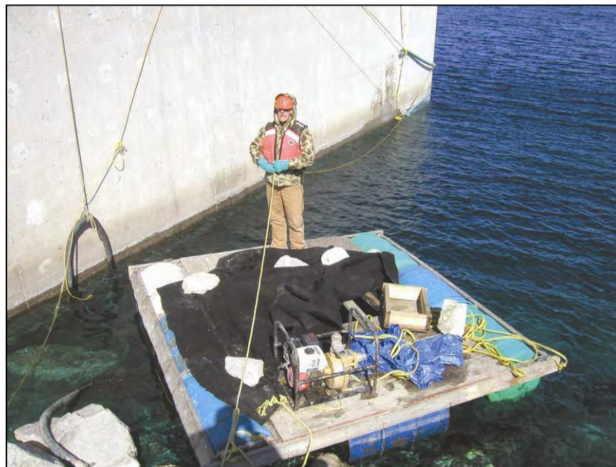
Figure A-129.—Barge used to monitor for grout blowout through foundation.
