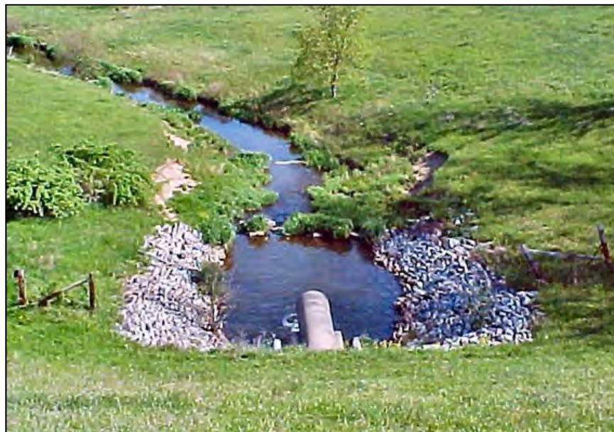
Figure 7.—A riprap-lined plunge basin downstream from a cantilevered pipe.
