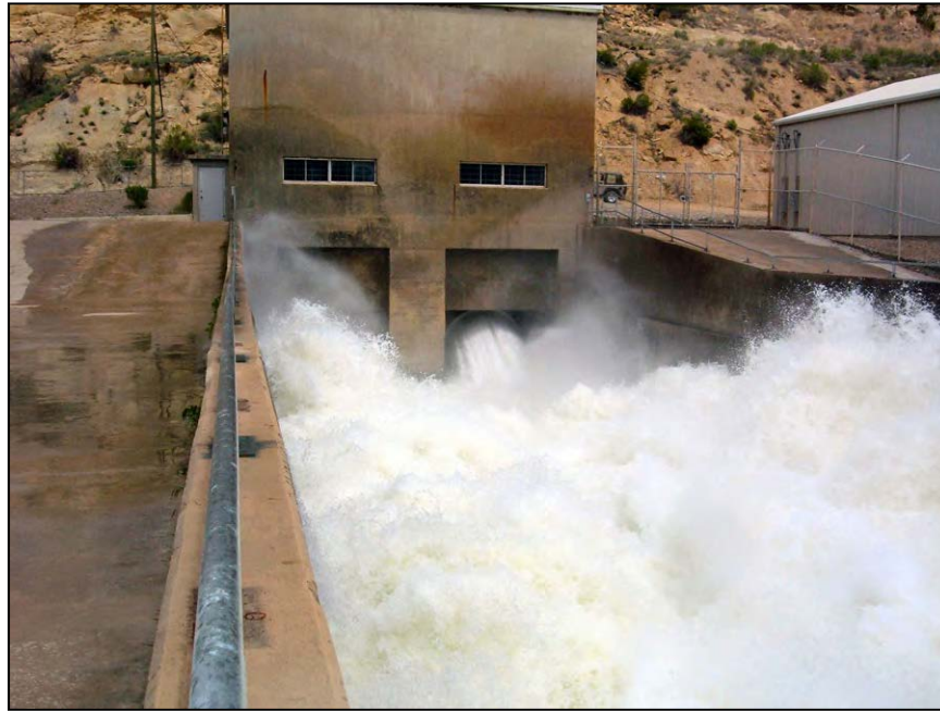
Figure A-55.—Both hollow-jet valves being operated at near full discharge capacity.
