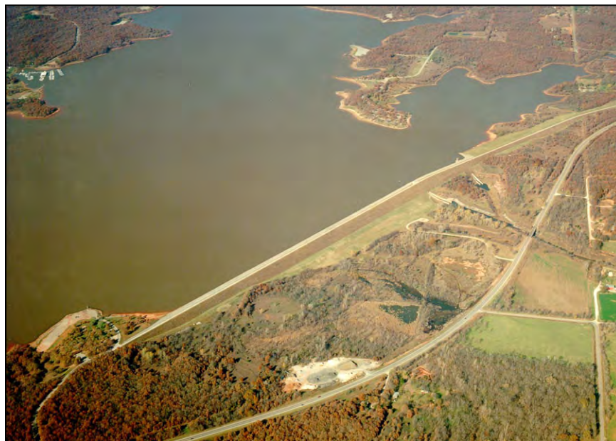
Figure A-59.—Aerial view of Norman Dam.
