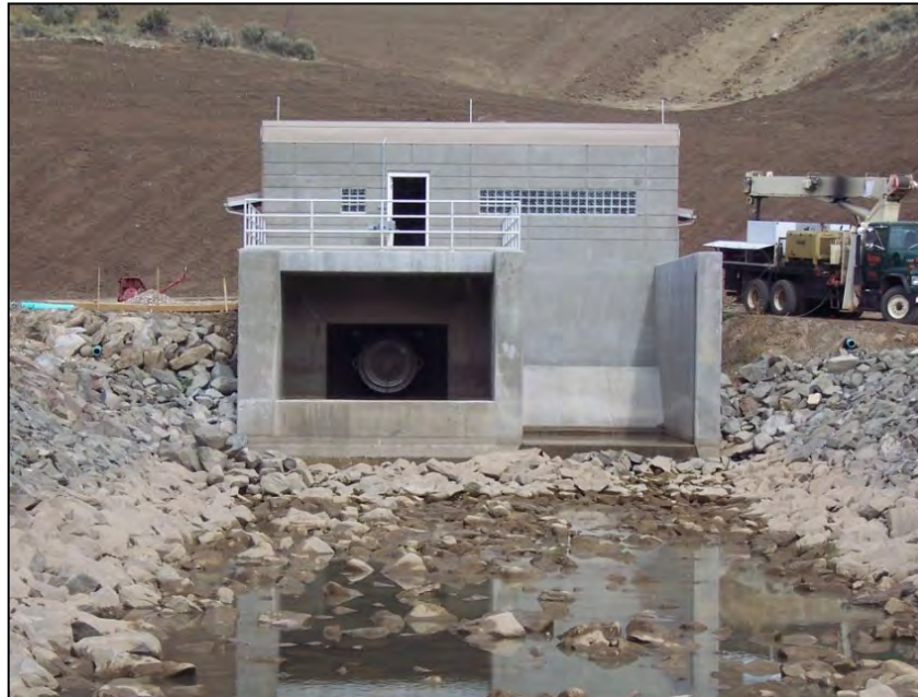
Figure A-19. —View of the completed energy dissipation structure for Elkhead Creek Dam with 42-inch diameter fixed-cone valve in background.
