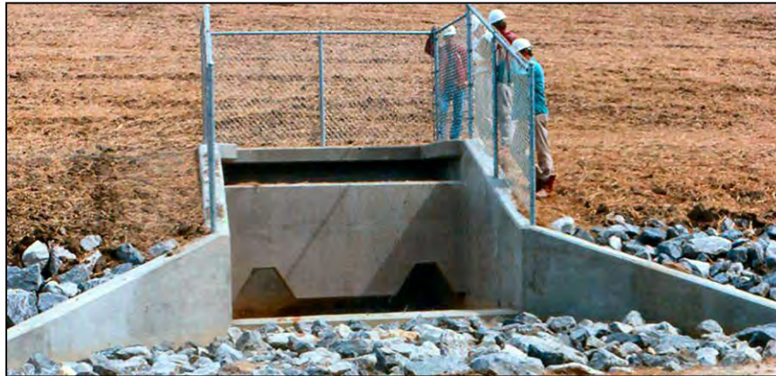
Figure 6.—A stationary baffle in an impact basin.
