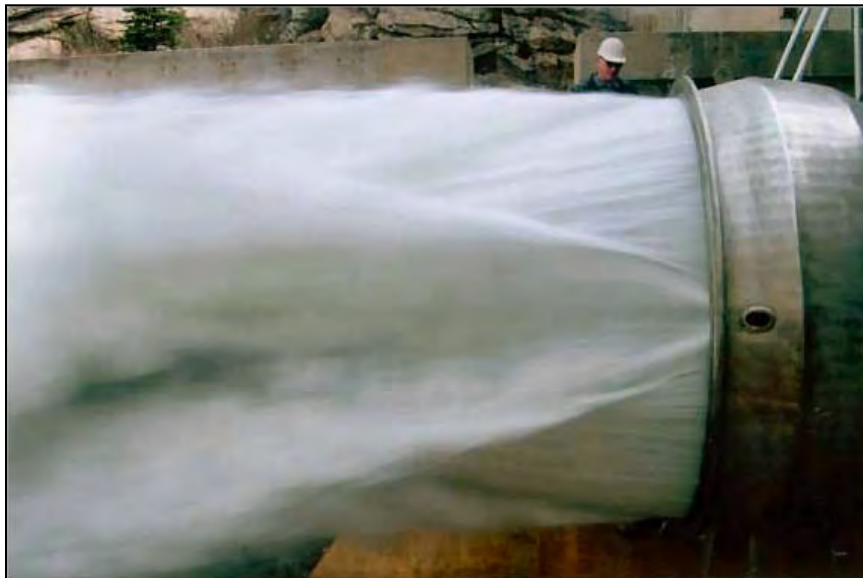
Figure 81.—48-inch diameter hooded fixed-cone valve discharge. Photo courtesy of URS Corporation and Denver Water Board.
