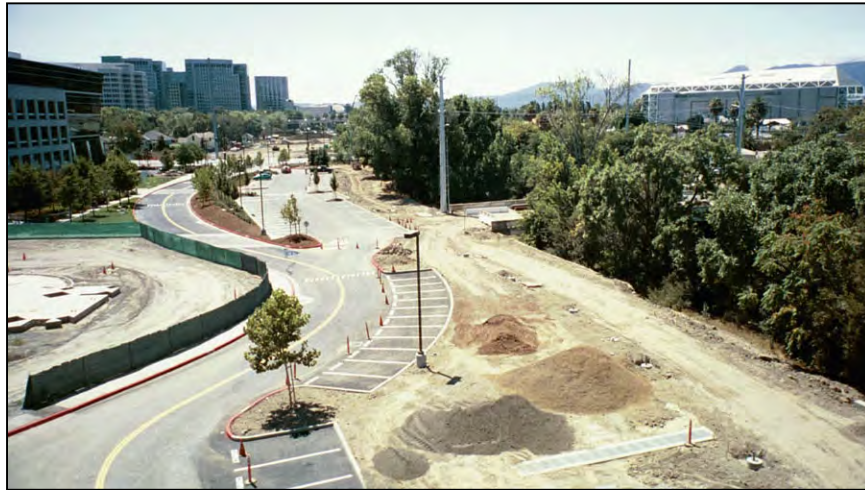
Figure A-29.—Culvert Under Sobrato Business Park.
