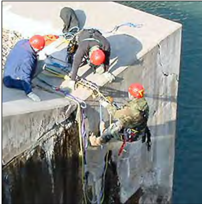
Figure 158.—A climbing team preparing to perform a wall inspection.
