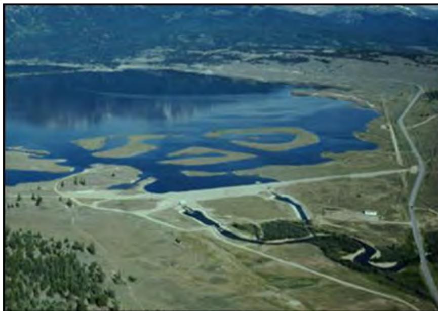
Figure A-103.—Aerial view of Twin Lakes Dam.
