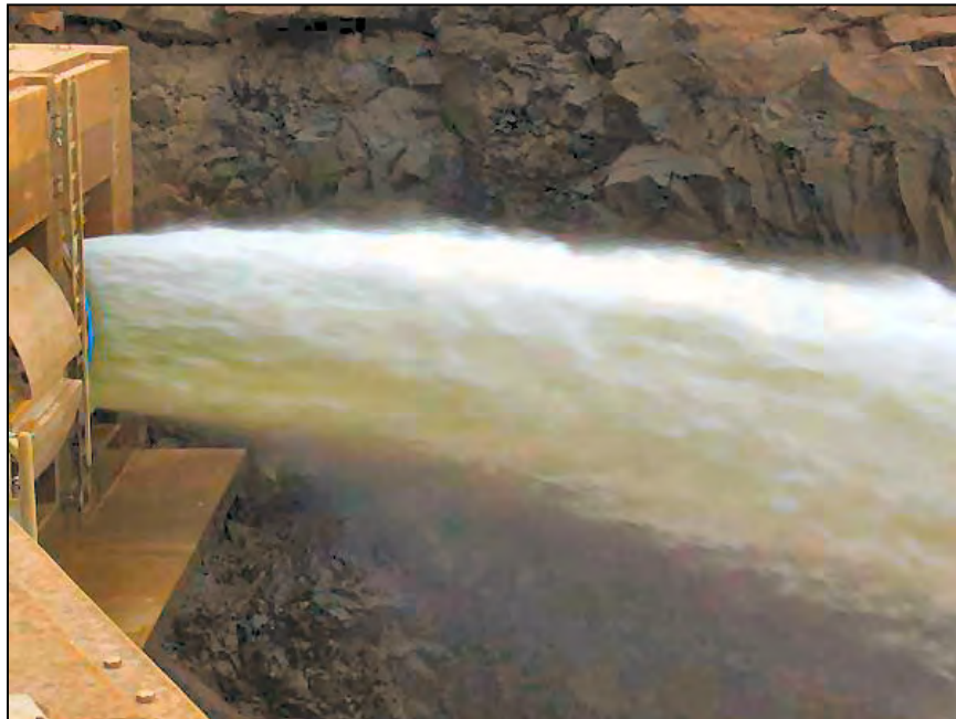
Figure 109.—68-inch diameter clamshell gate at 100-percent open.
