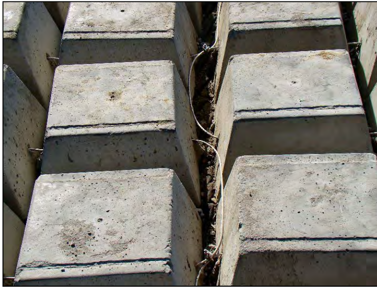
Figure 14.—Cable-tied concrete blocks.
