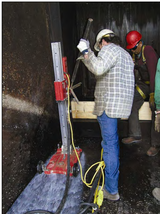
Figure A-126.—Drill crew drilling a hole in right bay of stilling basin.
