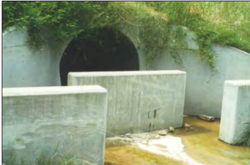
Figure 56.—A standard baffle basin.
