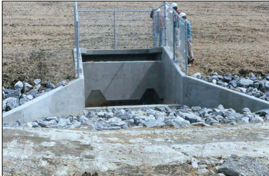
Figure 48.—Type VI impact basin with no flow being discharged.
