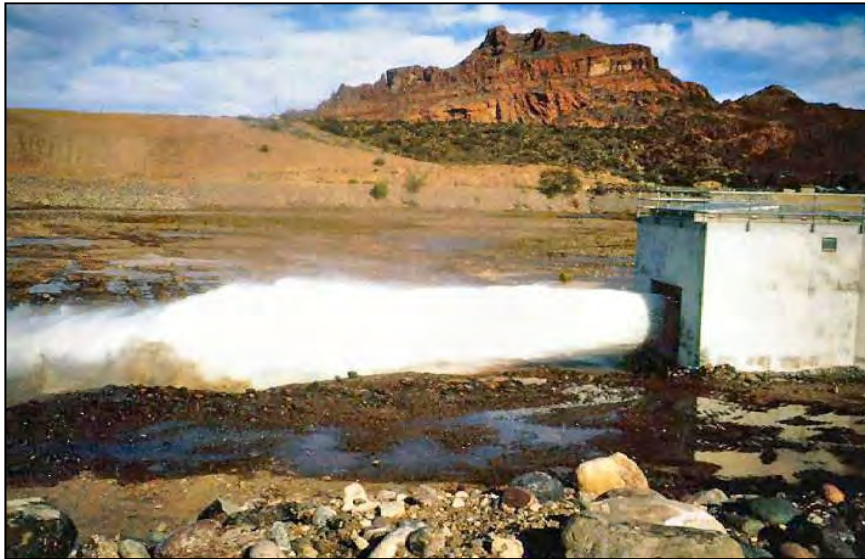
Figure 112.—78-inch diameter clamshell gate used for evacuation of a siphon.
