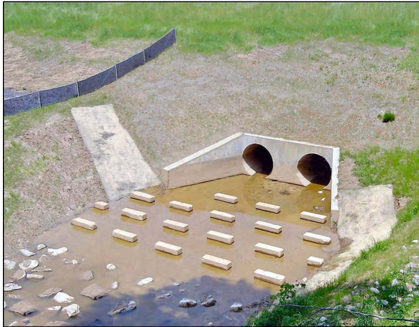
Figure 57.—Basin utilizing staggered rows of baffles.
