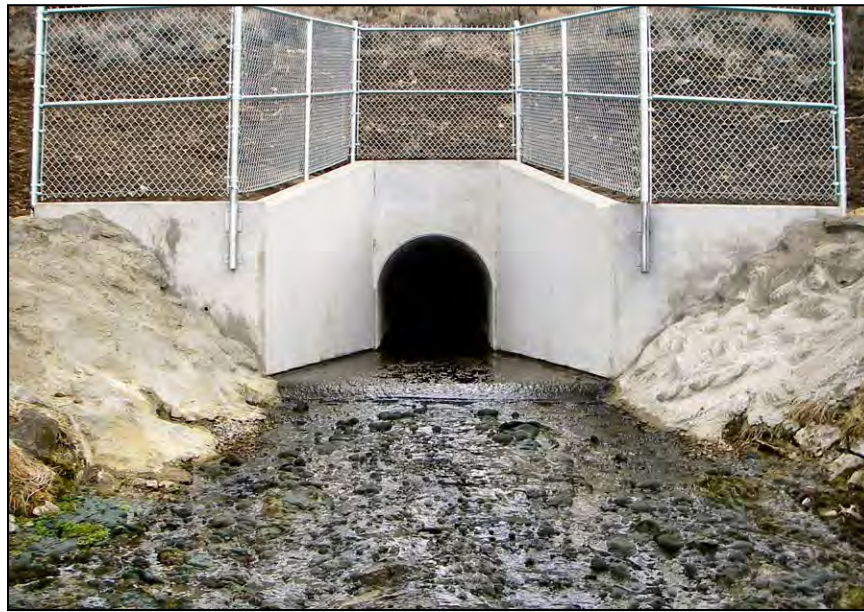
Figure 72.—A flared outlet transition.
