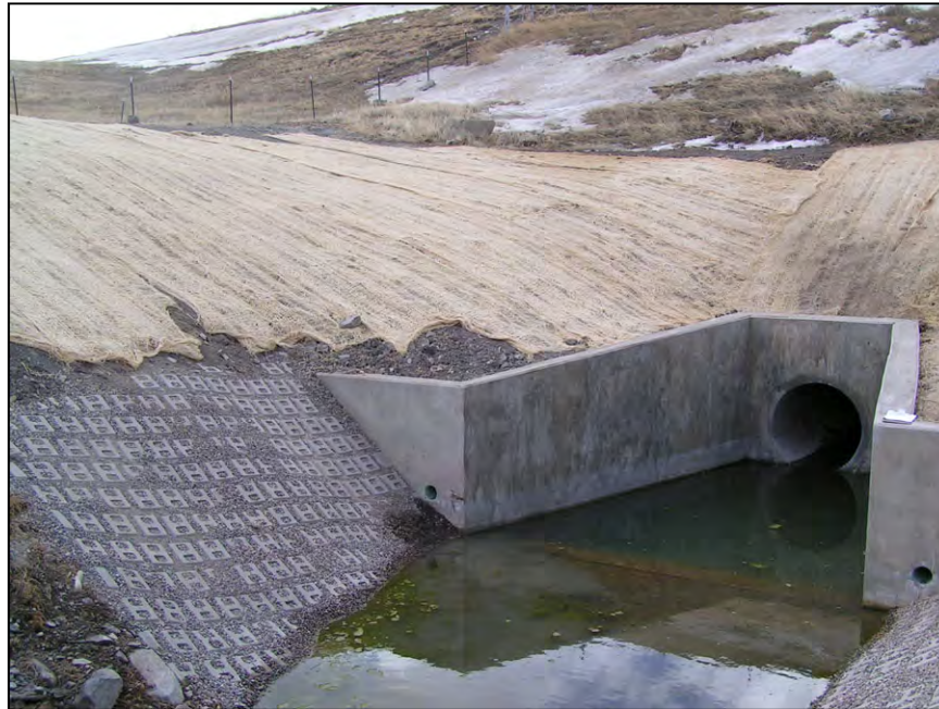
Figure A-58.—Replacement structure.
