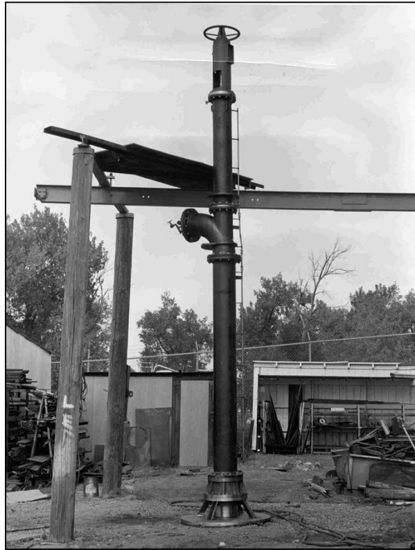
Figure 85.—A bottom discharge sleeve valve being fabricated.
