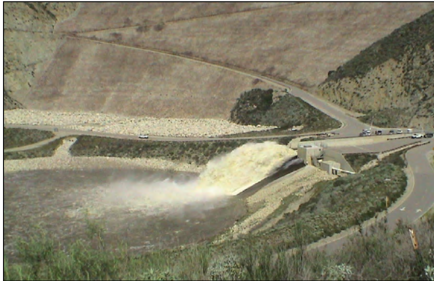
Figure A-89.—Plunge basin in operation at Seven Oaks Dam.
