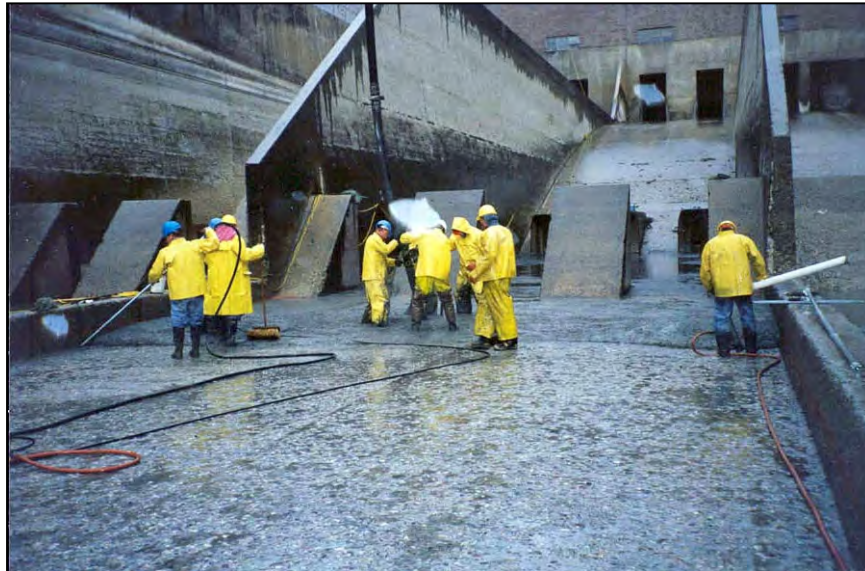
Figure A-73.—Closer view of concrete being placed.
