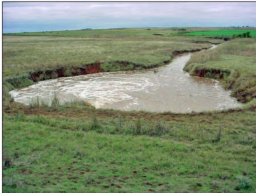
Figure 58.—Unlined plunge basin (view is looking downstream). This basin has been allowed to scour over time.
