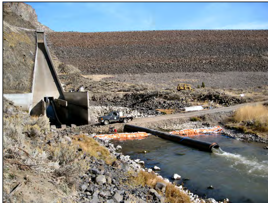
Figure 166.—Cofferdam constructed to keep the basin area dry for repairs.
