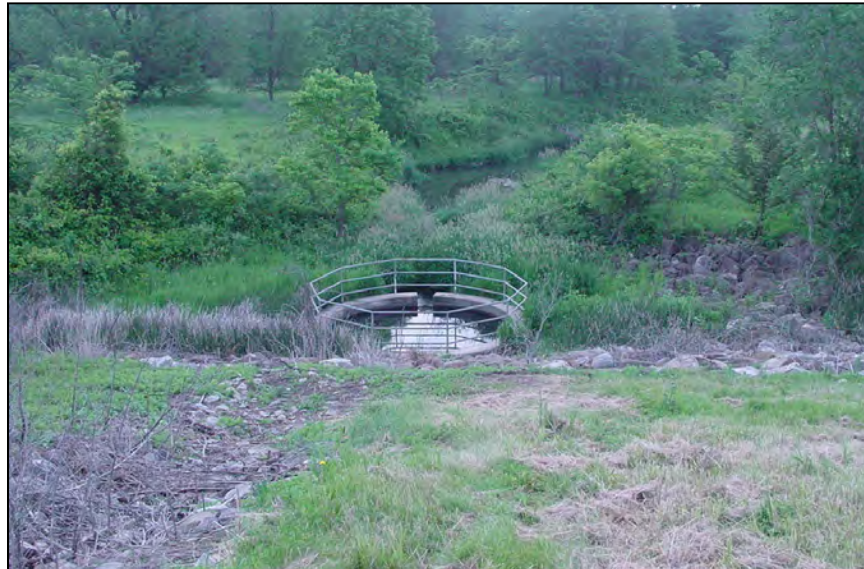
Figure 65.—Stilling well a at conduit outlet.
