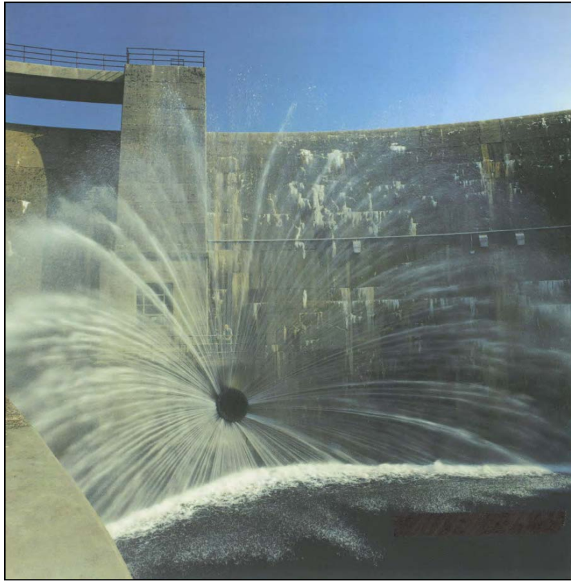
Figure 74.—Fixed-cone valve discharging at a small opening.
