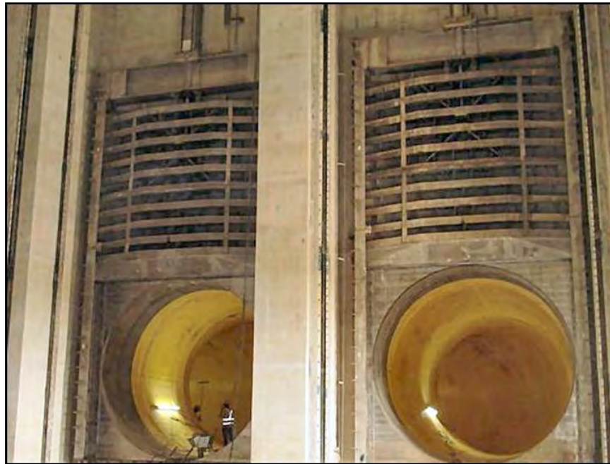
Figure 106.—Installation of large fabricated slide gates. Photo courtesy of Rodney Hunt Corporation.
