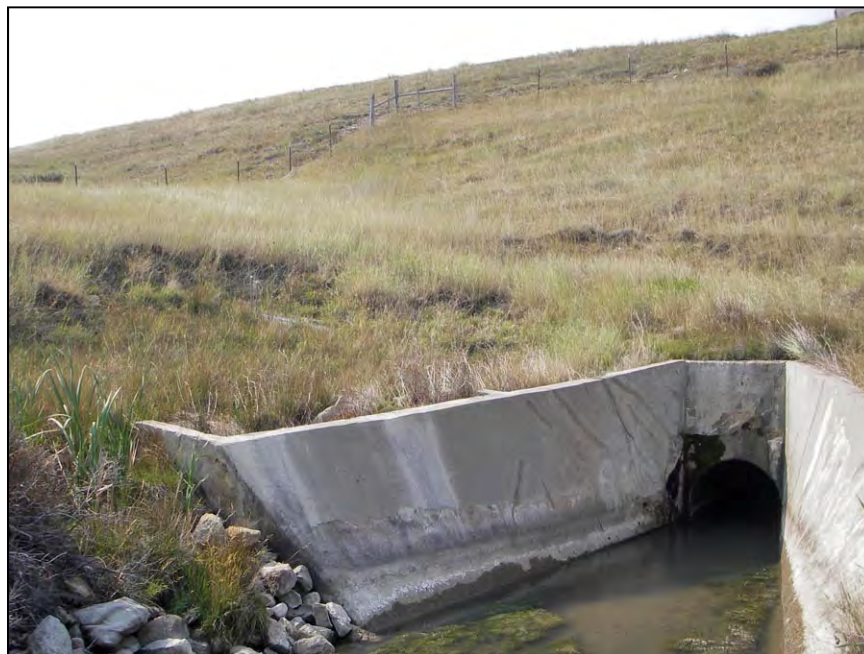
Figure A-56.—Original trapezoidal energy dissipator.
