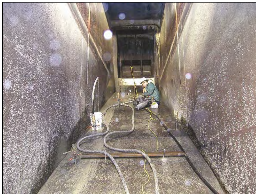
Figure A-128.—Grouting of the upstream chute.
