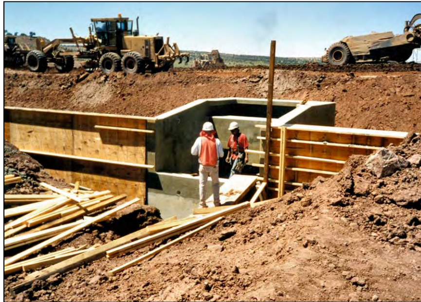
Figure A-26.—Construction crew installing forms for concrete placement of the stilling basin wingwalls.
