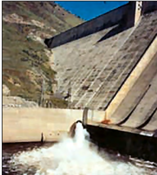
Figure 94.—Monovar valve used as a free discharge valve. Photo courtesy of Sapag.
