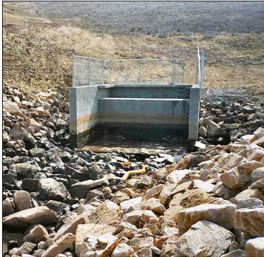
Figure 125.—Transitional riprap apron downstream for a type VI stilling basin to prevent scour.
