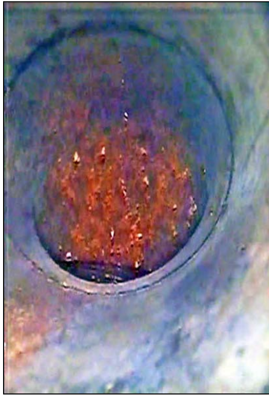
Figure A-108.—View of the first bend inside Underdrain No. 1 (rightmost drain) in the outlet works stilling basin. Image was taken from pipe inspection video.
