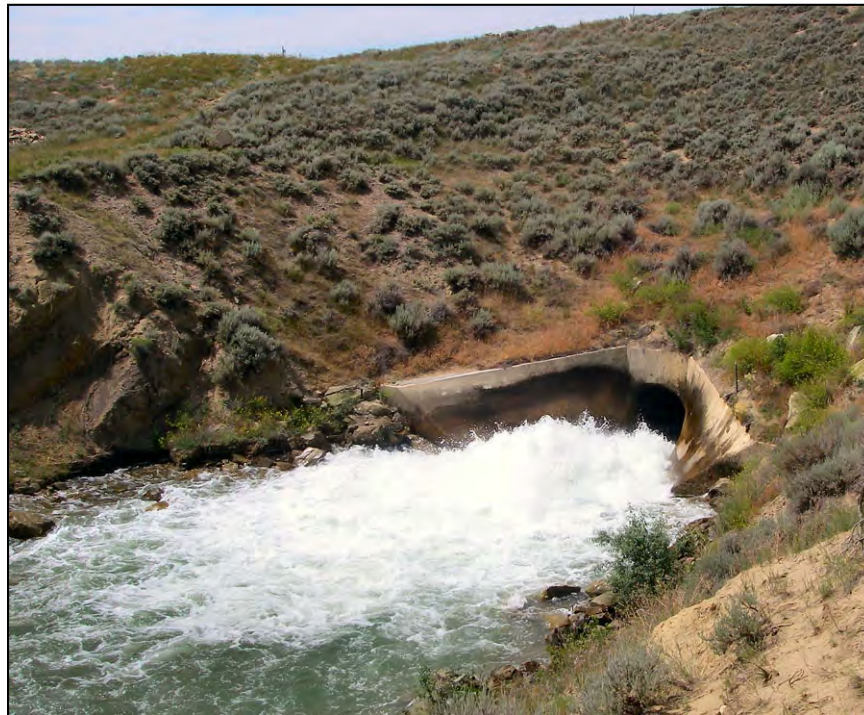
Figure 71.—7.5-foot horseshoe conduit discharging into an outlet expansion with a depressed floor. Downstream channel armoring has also been provided.
