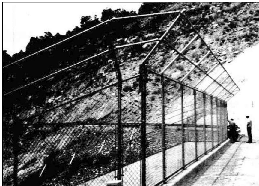
Figure 180.—Inclined fencing to reduce damage from vandalism (Reclamation, 1993, p. 1).
