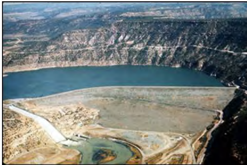
Figure A-53. —Aerial view of Navajo Dam. The hollow-jet-valve outlet works basin is located next to the spillway stilling basin.
