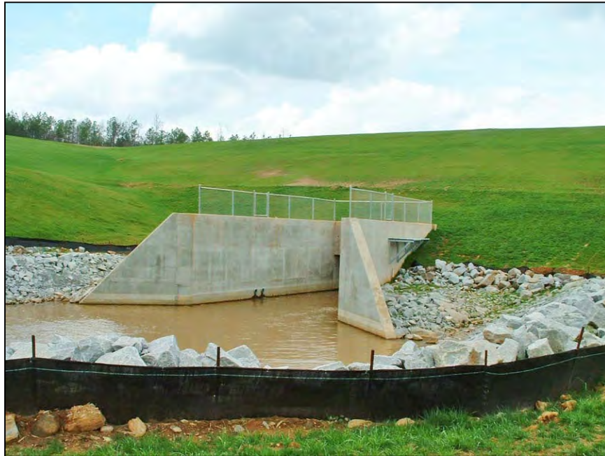
Figure 175.—Fencing installed along the tops of the stilling basin walls.
