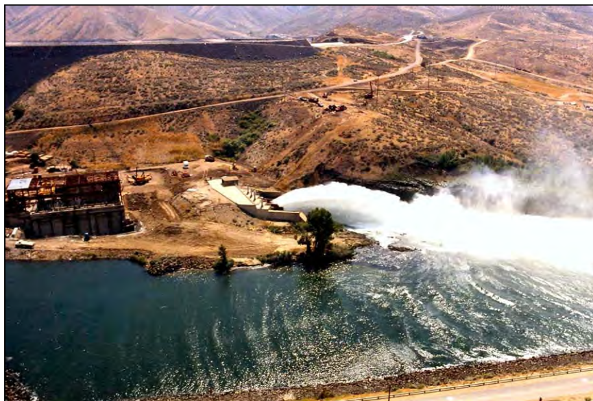
Figure A-44.—Discharge emerging from flip bucket operations.
