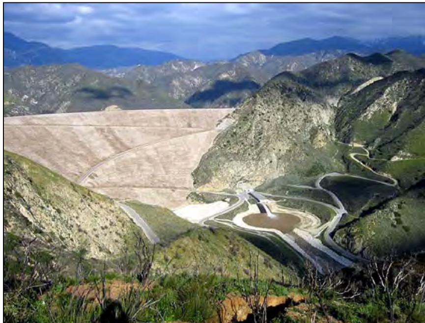
Figure A-84.—Seven Oaks Dam.
