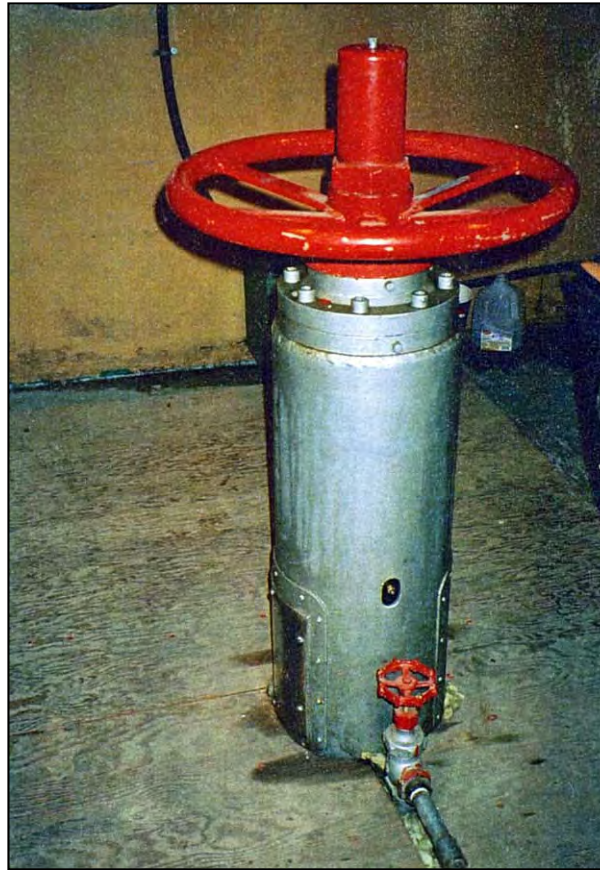
Figure A-3.—Handwheel control for sleeve valve. The handwheel requires 3\frac{3}{4} turns to fully open the valve from the closed position.
