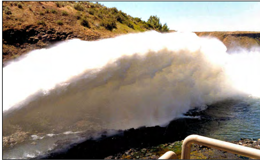
Figure A-45.—High velocity flow being directed downstream into the plunge basin.
