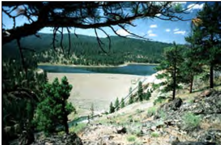
Figure A-48.—Mason Dam as seen from the left abutment.
