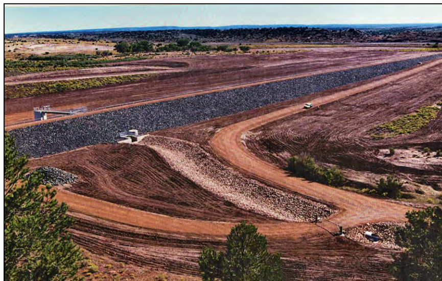
Figure A-25.—Overall view of completed dam modifications from downstream right abutment. The outlet works stilling basin is located in the left center of the figure.
