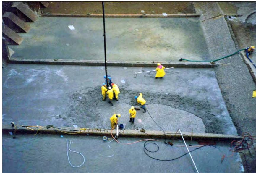
Figure A-72.—Concrete being pumped for placement at floor.
