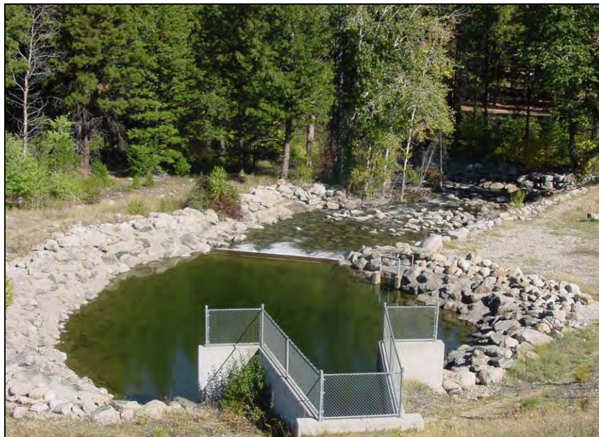
Figure 10.—Conduit outlet expansion.
