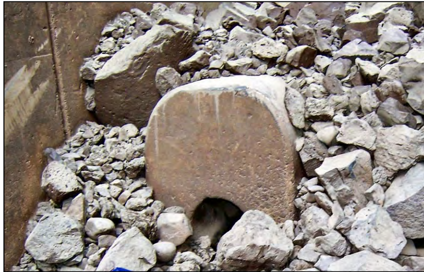
Figure 153.—Debris deposited around a chute block.
