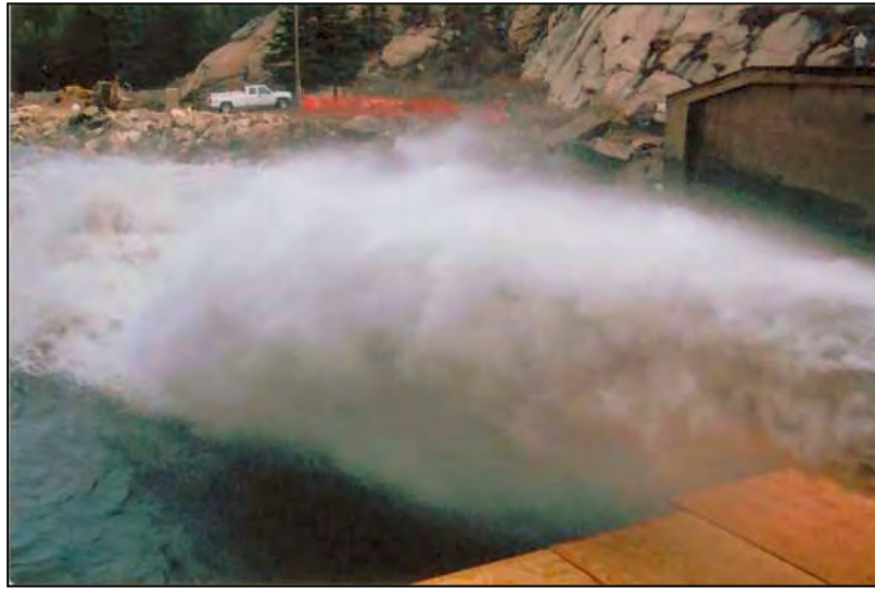
Figure 82. —48-inch diameter hooded fixed-cone valve discharge. Photo courtesy of URS Corporation and Denver Water.
