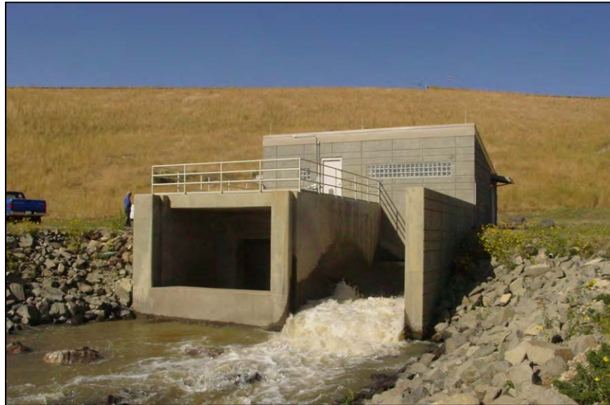
Figure A-23.—View of 18-inch diameter jet-flow gate discharging at about 50 to 70 ft 3 /s (near maximum discharge capacity).
