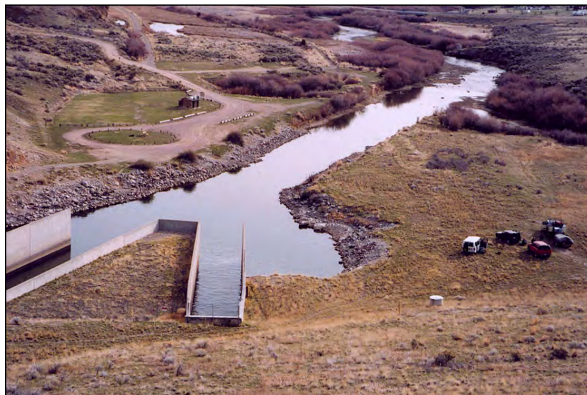
Figure A-9.—View looking downstream from top of dam with outlet works stilling basin in middle and spillway stilling basin to the left.
