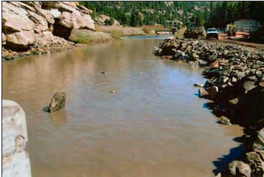
Figure 84. —Erosion of riprap downstream from a 48-inch diameter hooded fixed-cone valve. Photo courtesy of URS Corporation and Denver Water Board.
