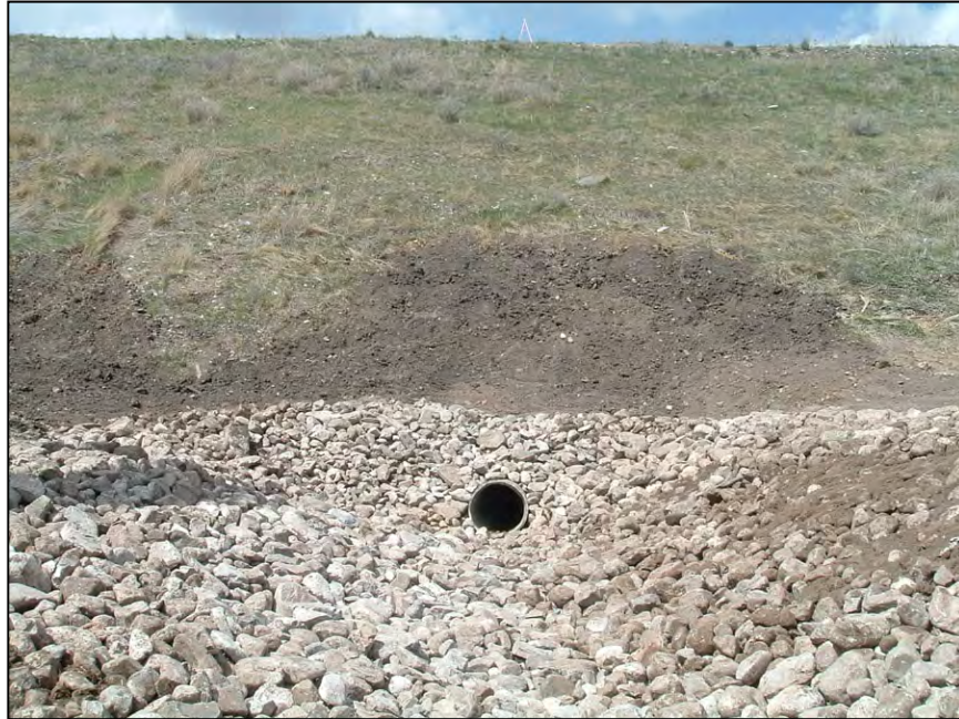
Figure 122.—A riprap apron used for erosion protection.
