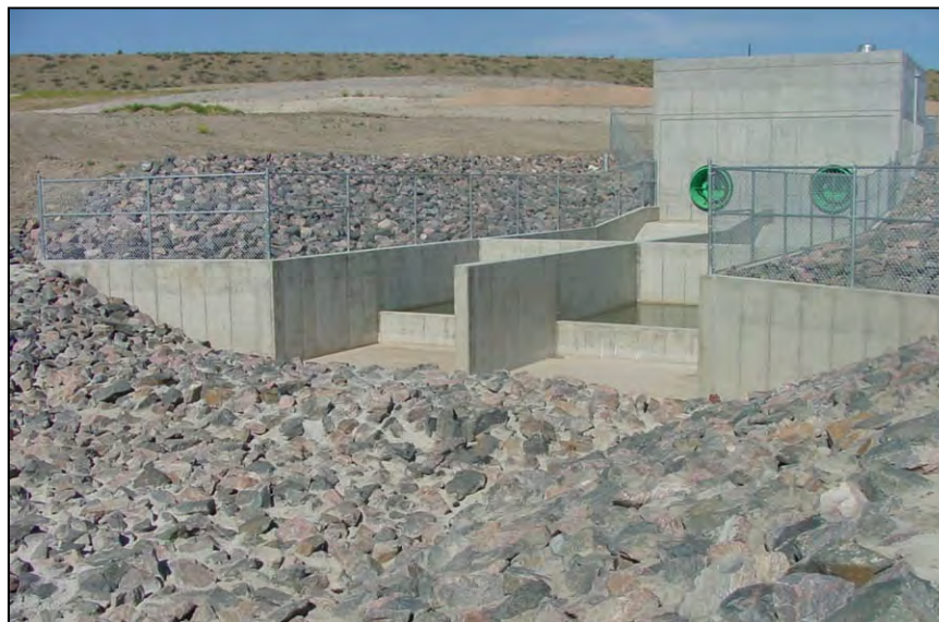
Figure A-97.—View of completed stilling basin for the new outlet works at the stream release facility at Standley Lake Dam.
