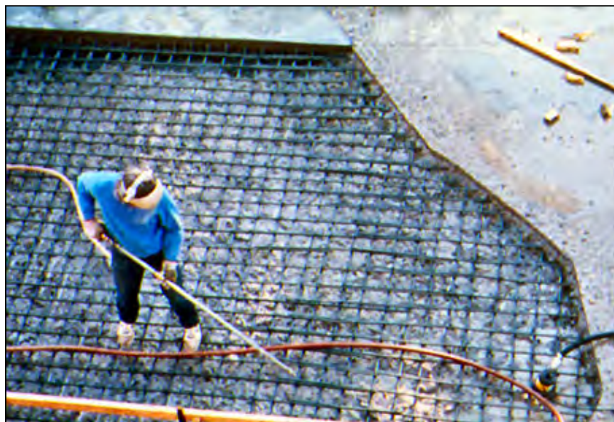
Figure 172.—Blowing compressed air over the surface of the concrete to remove excess moisture.
