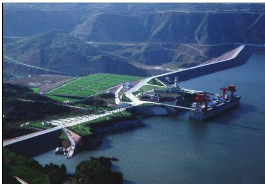
Figure A-130.—Aerial view of Xiaolangdi Dam.
