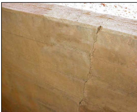
Figure 149.—Vertical crack in wall. Figure 150.—Loss of joint filler in a wall joint.
