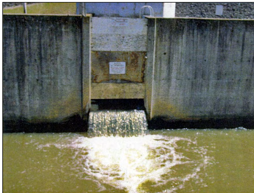
Figure A-5.—Outlet works discharge enters the spillway stilling basin through an opening in the right wall.
