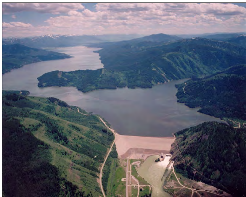
Figure A-67.—Aerial view of Palisades Dam.
