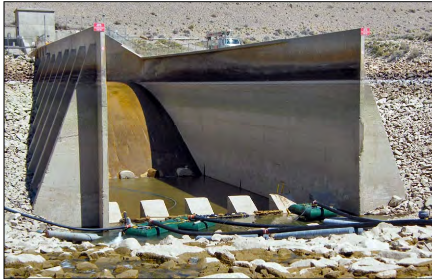
Figure 24.—Type II stilling basin with counterforted walls. The basin has been unwatered for repairs.
