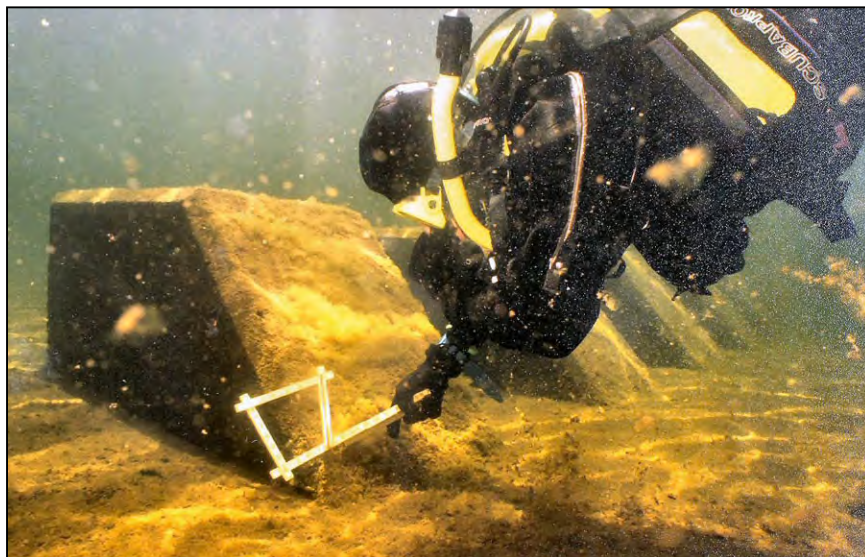
Figure 156.—A diver inspecting a baffle block.
