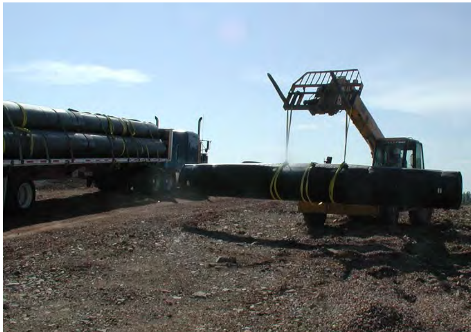
Figure 6.2.—Photograph showing proper offloading of geotextile product rolls. Cloth slings rather than the forks of the lift are used to properly unload this delivery.
