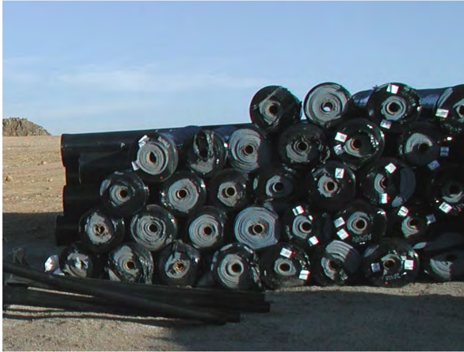
Figure 6.3.—Photograph of geotextile storage. A layer of fine-grained soil was placed in the storage area to avoid placing the rolls directly on the rocky soil which is visible in the left side of the photograph. Damage to the ends of the protective wrappers is evident, the inspector required these rolls to be covered by a tarp to prevent contamination by dust and to avoid degradation from prolonged UV exposure.
