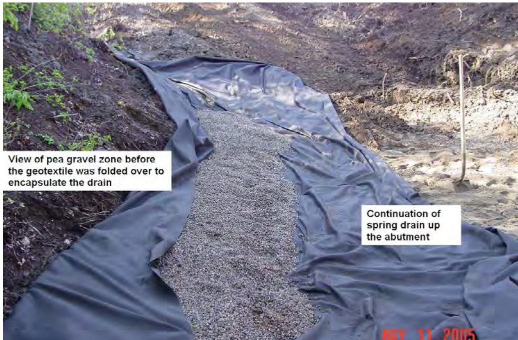
Figure 3 – Pea gravel drainage zone prior to encapsulating it in the geotextile.
