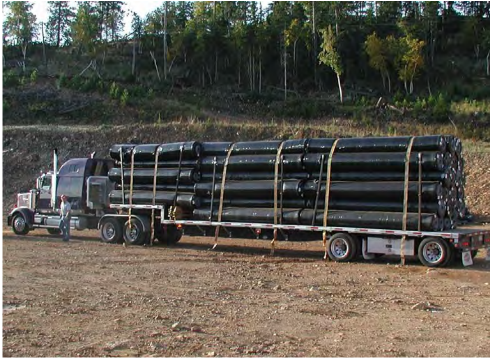
Figure 6.1.—Photograph of a truck delivering geotextile rolls to a construction site. The tie down straps at the front of the truck are intruding into and have distorted the shape of the top roll. This roll must be carefully examined to verify that it has not been damaged during transport.
