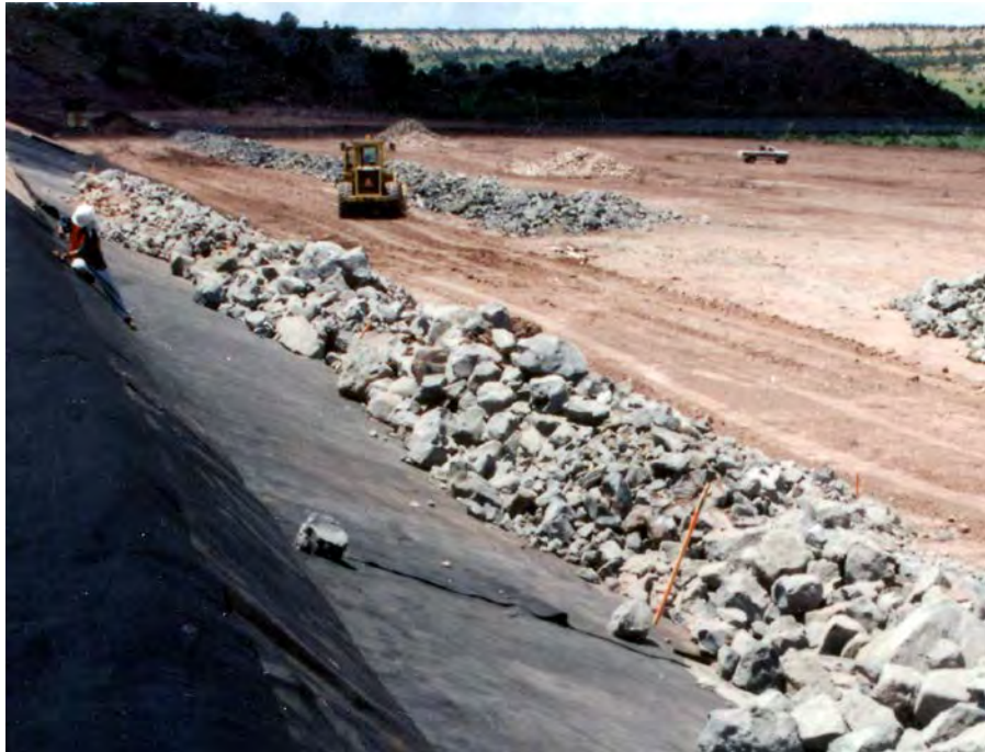
Figure 6.12.—Photograph showing riprap placed directly onto a geotextile. The slope height that can be covered by this method is limited by the reach of the equipment.
