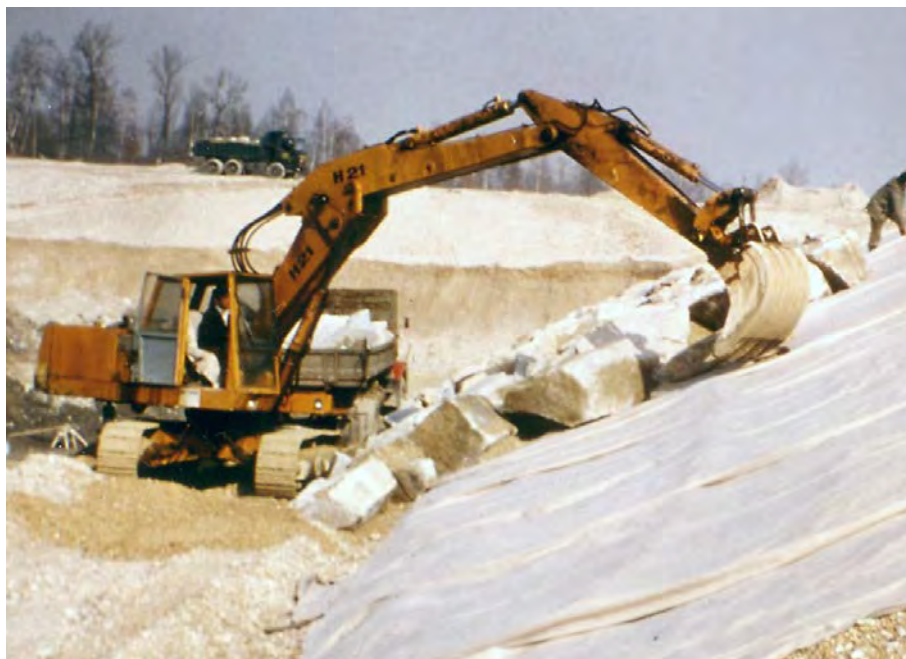
Figure 6.12.—Photograph showing riprap placed directly onto a geotextile. The slope height that can be covered by this method is limited by the reach of the equipment.
