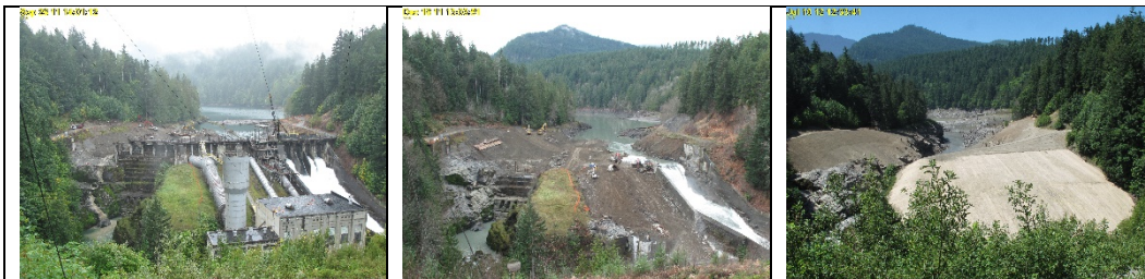
Figure 35.—Elwha Dam on the Elwha River prior to just to dam removal in 2011 (left), during dam removal in 2012 (center), and after dam removal in 2012 (right).
