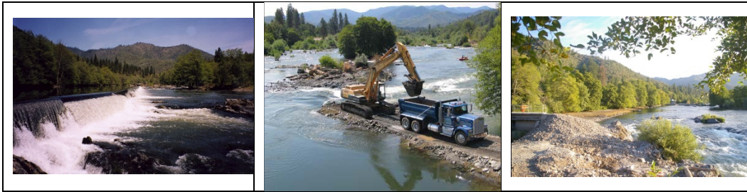
Figure 32.—Gold Hill Dam on the Rogue River prior to dam removal in 1999 (left), during dam removal in 2008 (center), and after dam removal in 2008 (right).
