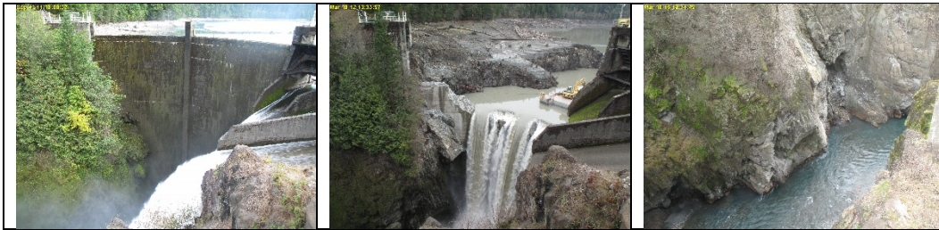
Figure 37.—Glines Canyon Dam on the Elwha River prior to just to dam removal in 2011 (left), during dam removal in 2012 (center), and after dam removal in 2015 (right).
