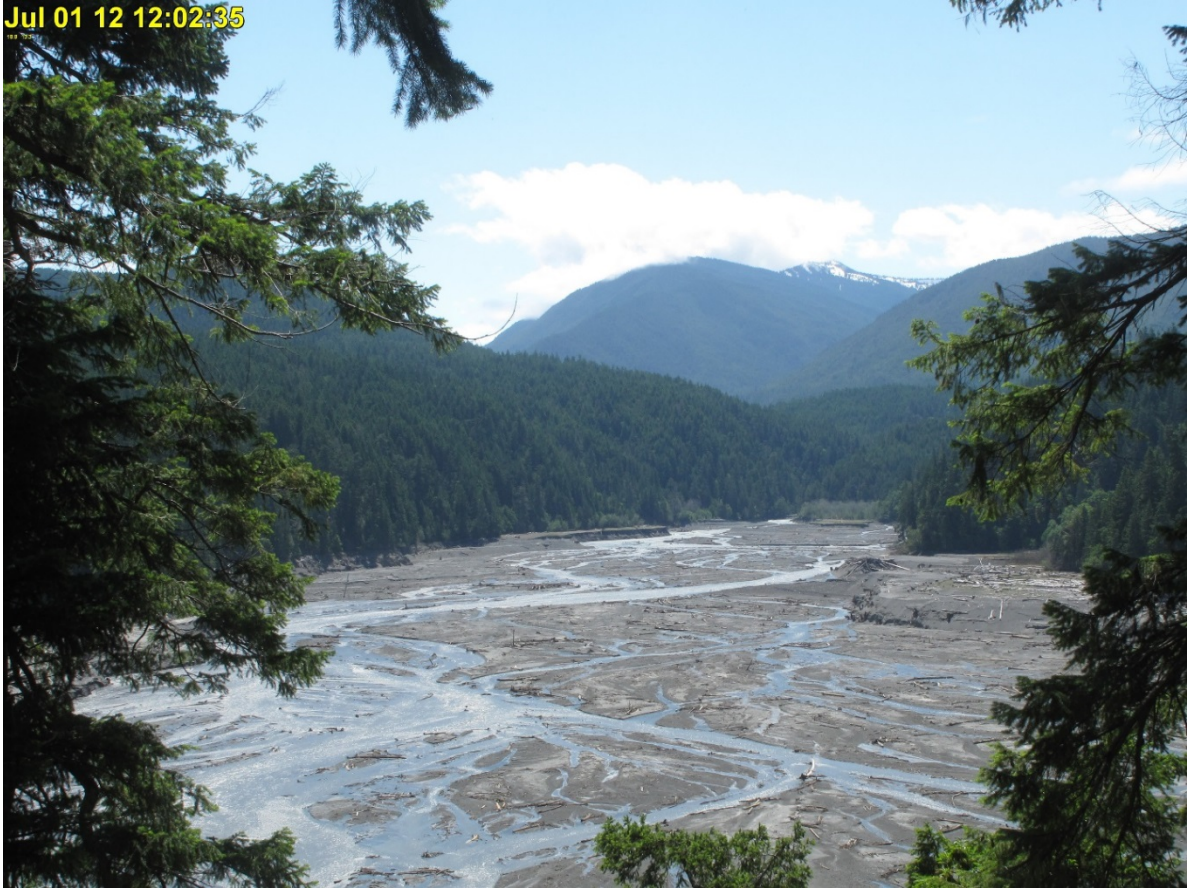
Figure 26.—Looking upstream at extensive lateral erosion of Lake Mills delta (upper coarse layer) near Port Angeles, WA less than 1 year after phased dam removal began.
