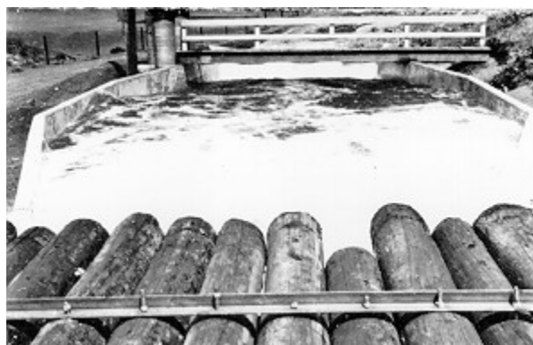
Figure 5-4 -- Turbulence and waves in a Parshall flume produced by an outlet works stilling basin. The log raft failed to quiet the flow.
