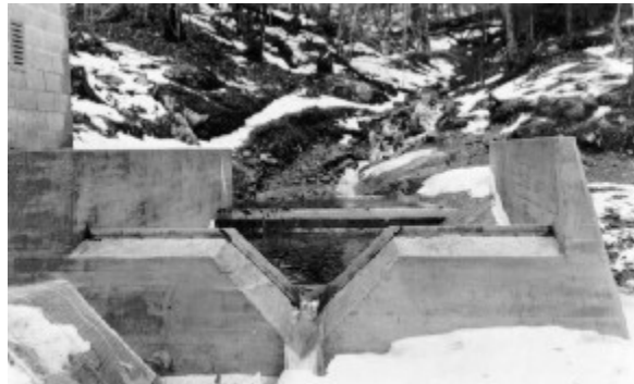
Figure 7-10 -- Compound weir with 90-degree notch and suppressed rectangular crest used by U.S. Forest Service.
