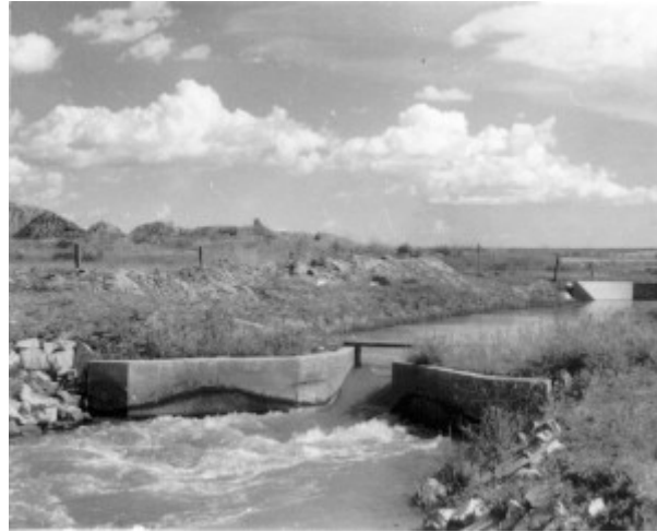
Figure 8-2 -- Four-foot, short-form Parshall flume, discharging 62 \text{ ft}^3/\text{s} under free-flow conditions. Scour Protection is needed for this much drop.
