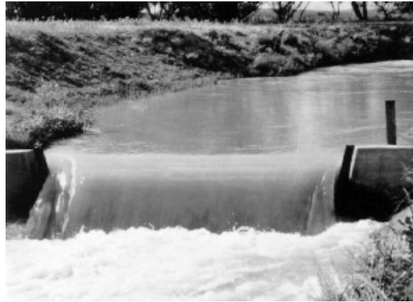
Figure 7-2 -- Cipolletti weir operating with full contractions at the end and on the crest.
