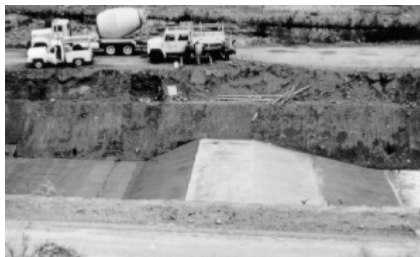
(a) Long-throated flume (broad-crested weir) under construction.
