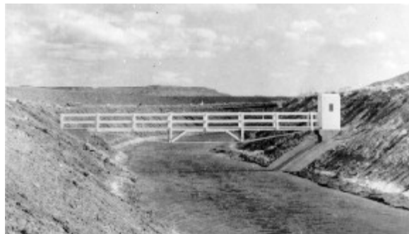
Figure 10-1 -- Current-meter station on a canal, viewed from upstream. Current-meter measurements are taken from the bridge, and the sheltered stilling well houses an automatic water-stage recorder.
