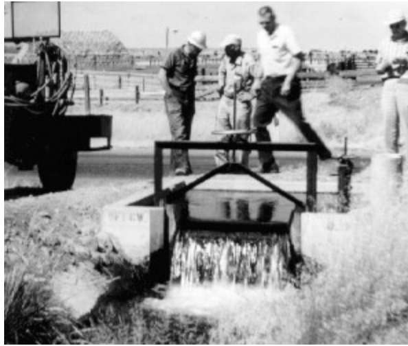
Figure 7-14 -- Adjustable Cipolletti weir in a division box.
