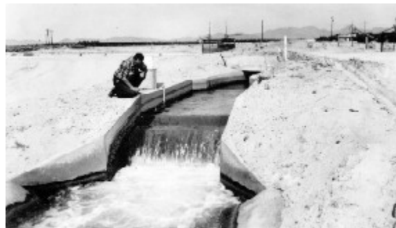
Figure 7-3 -- Suppressed rectangular weir at a canal drop.
