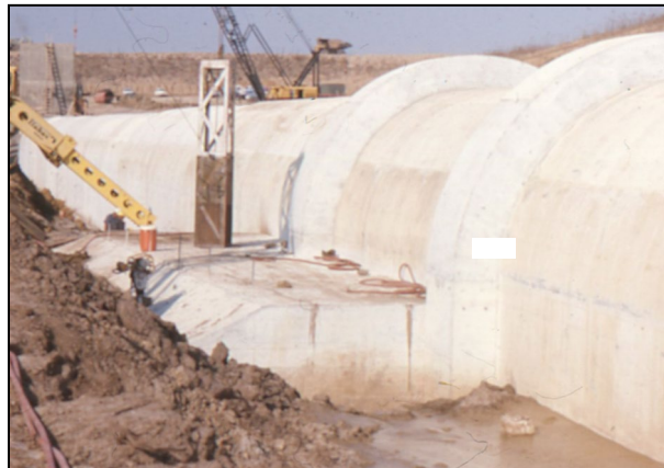
Portion of concrete plug along conduit
