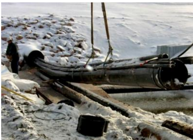
Photo 2: Installing HDPE Liner pipe. 2
