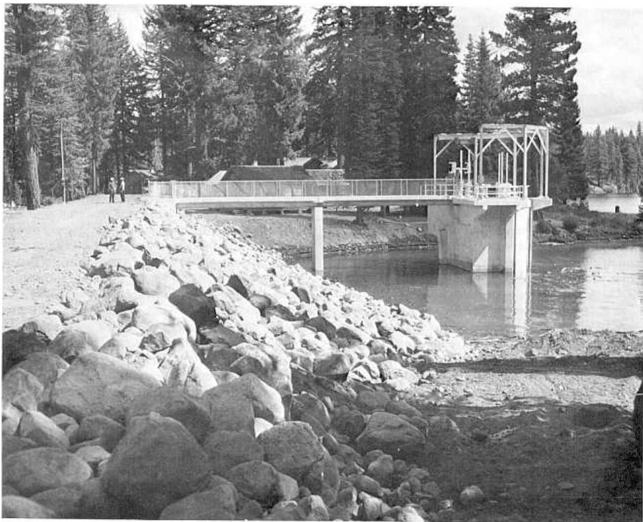
Figure 4-1.—Crescent Lake Dam, a small earthfill storage dam on Crescent Creek in Oregon. 806-126-92.
