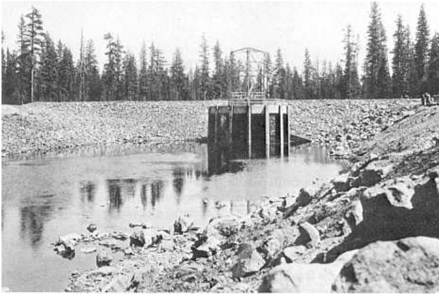
Figure 6-1.—Upstream face of dam and fishscreened inlet structure. Crane Prairie Dam on the Deschutes River in Oregon.
