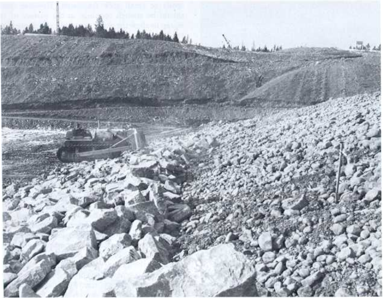
Figure 6-48.—Placing riprap on an upstream slope. Meeks Cabin Dam, Wyoming. P415-432-720.
