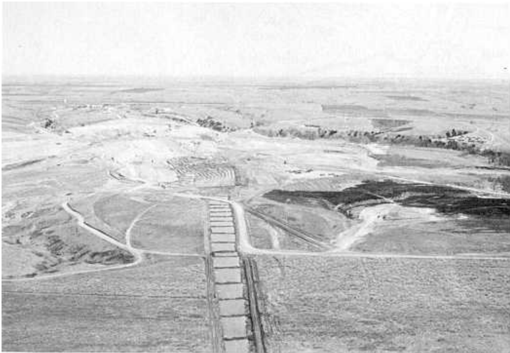
Figure 6-37.—Ponding on foundation of Medicine Creek Dam. 404-1227B.
