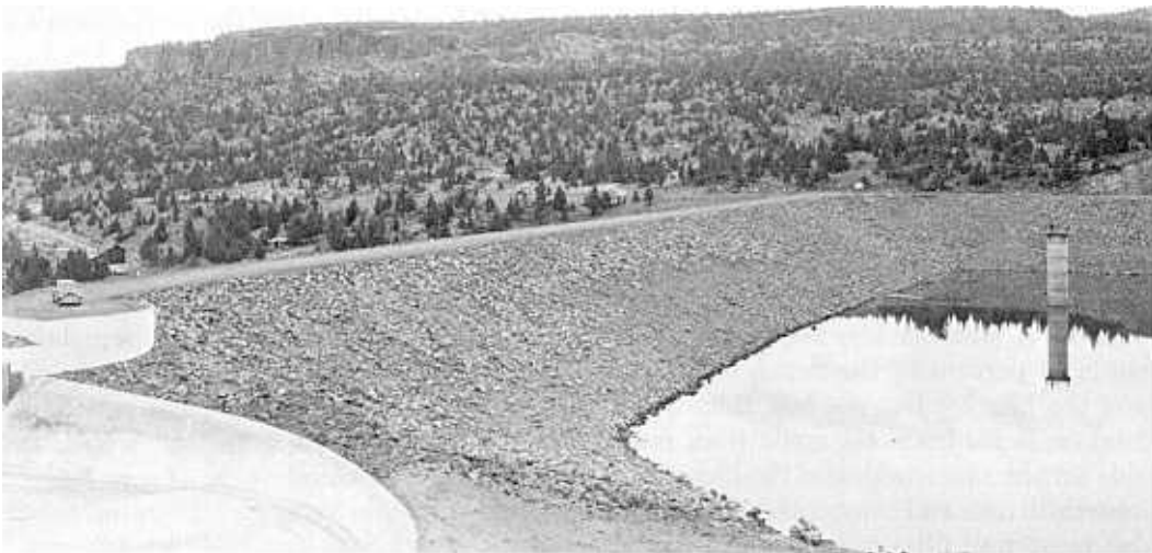
Figure 6-22.—Upstream slope of Ochoco Dam.
