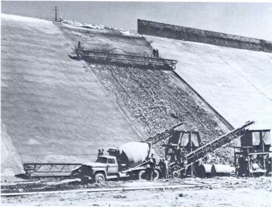
Figure 7-15.—Placement of shotcrete on the upstream face of Taum Sauk Dam, Missouri. (Union Electric Co. photograph). 288-D-2883.
