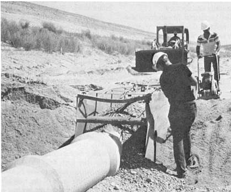
Figure 6-26.—Toe drain construction at Calamus Dam, Nebraska. P801-D-81041.
