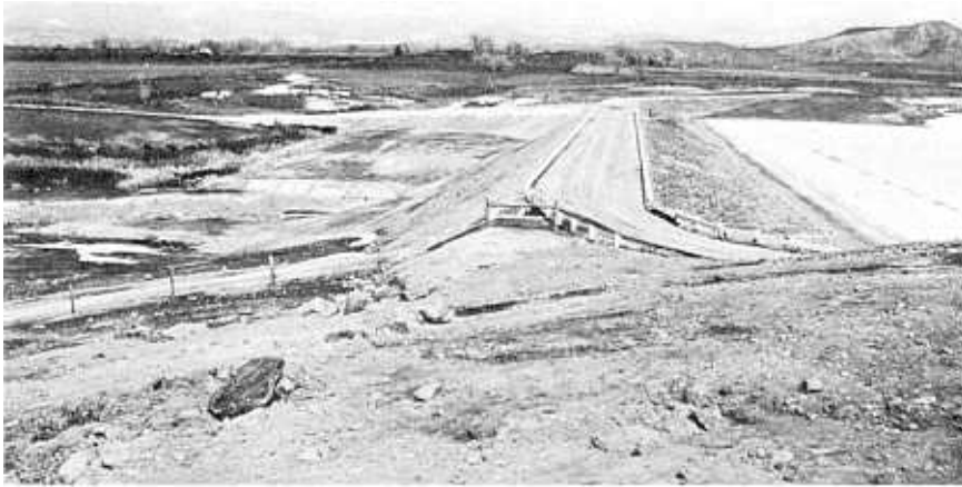
Figure 6-2.—Fruitgrowers Dam, an earthfill storage dam at an offshore location in Colorado.
