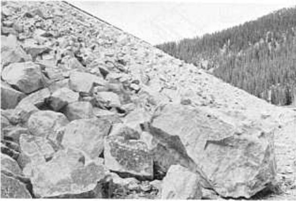
Figure 7-6.—Granite rockfill on downstream face of Montgomery Dam, Colorado. CH-520-150.
