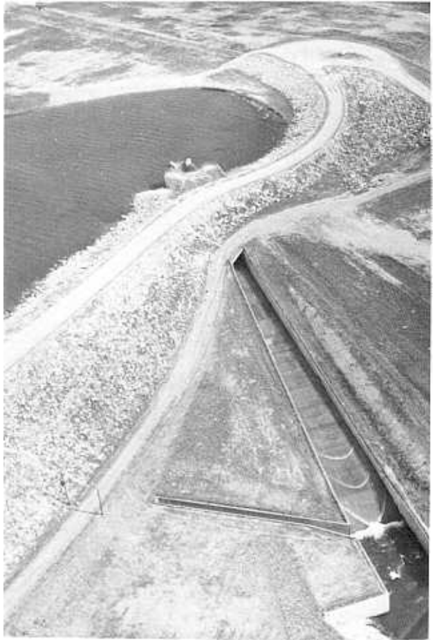
Figure 9-9.—Aerial view of service and auxiliary spillways. (Same spillway shown on figs. 9-7 and 9-8). 288-D-2897.
