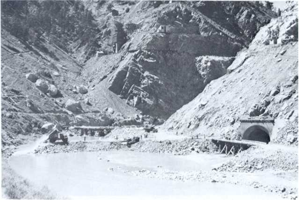
Figure 11-5.—Diversion adit and upstream cofferdam at Seminole Dam.
