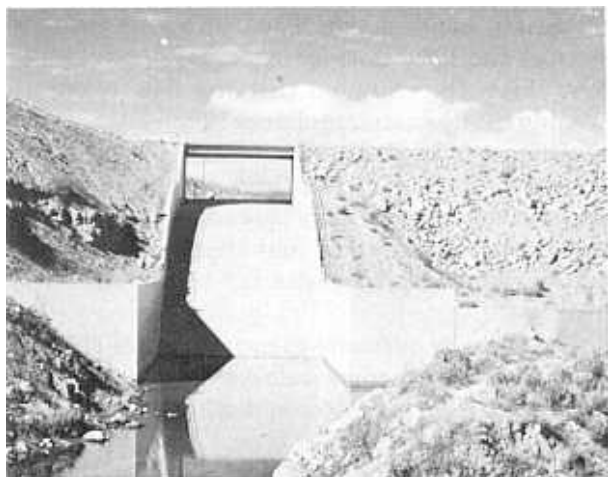
Figure 9-14.—Chute spillway for Scofield Dam, Utah. 288-D-2901.
