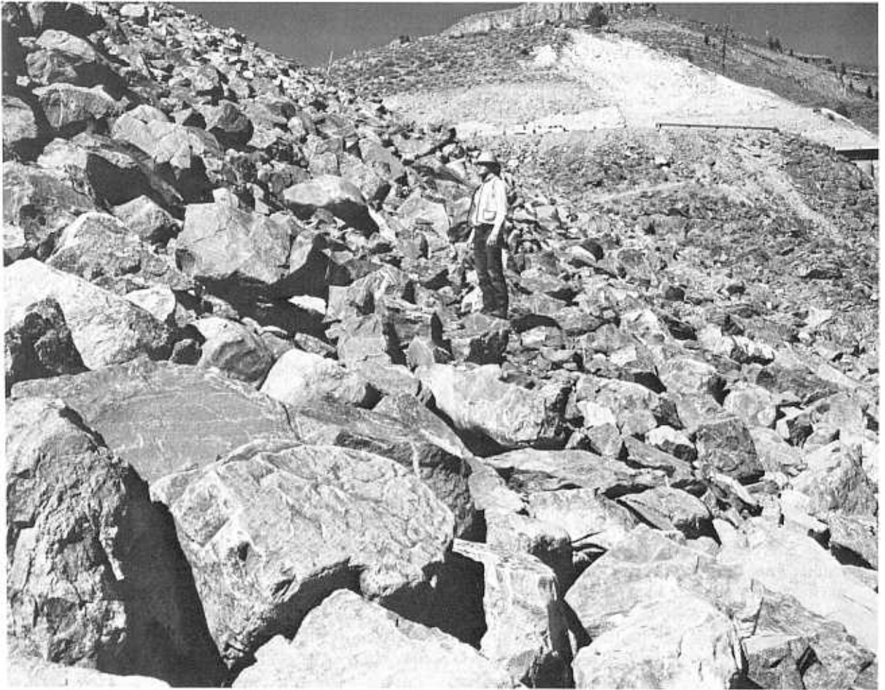
Figure 6-50.—Completed riprap slope protection on upstream face of Blue Mesa Dam, Colorado. P662A-427-10496NA.
