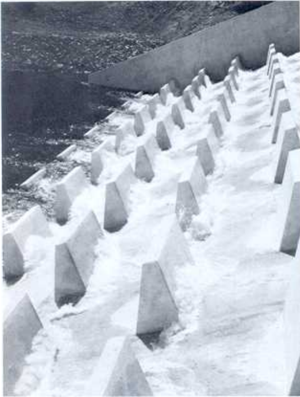
Figure 9-17.—Baffled chute drop spillway. Conconully Dam, Washington. The flow shown passing over the spillway is about 50 ft 3 /s. P21-141-178NA.
