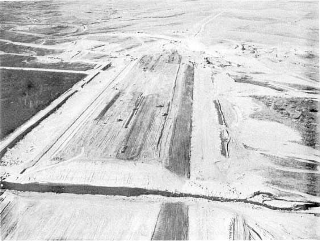
Figure 11-8.—Temporary diversion channel through an earthfill dam. Bonny Dam. 414-289C.
