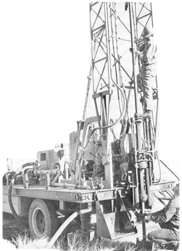
Figure 5-52.—Diamond-core drill rig used in exploration of a dam foundation. E-2255-4NA.
