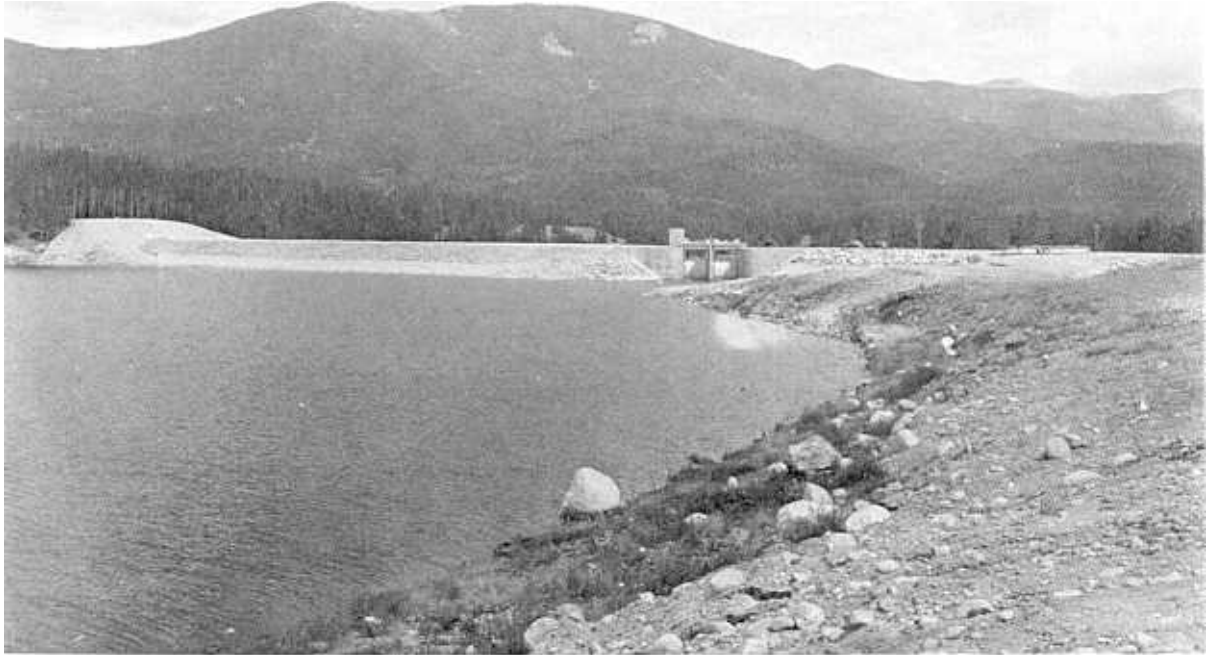
Figure 6-3.—Shadow Mountain Dam, an earthfill structure on the Colorado River in Colorado. Constructed as part of a large transmountain diversion scheme. SM-175-CBT.
