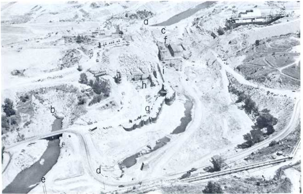
Figure 11-4.—Diversion of the American River during construction of Folsom Dam and Powerplant. (Corps of Engineers and Bureau of Reclamation). AR-1627-CV.
