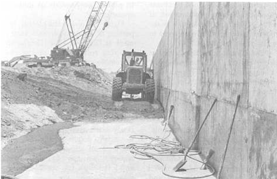
(b) Zone 1B against outlet conduit. P801-D-81038.
