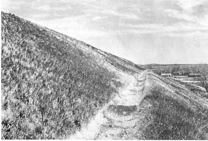
Figure 6-56.—Downstream slope of Belle Fourche Dam protected by grass. 288-D-2938.
