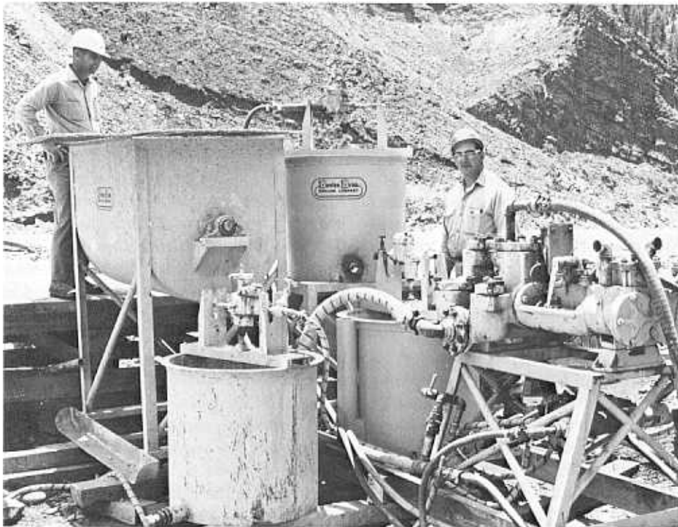
Figure 6-11.—Grouting plant used at Ruedi Dam, Colorado. P382-706-1134NA.
