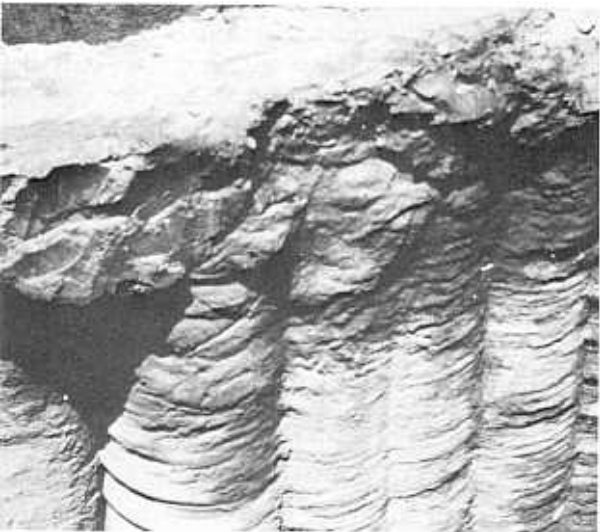
(B) Finished wall. (Intrusion-Prepakt Co.). 288-D-2876.
