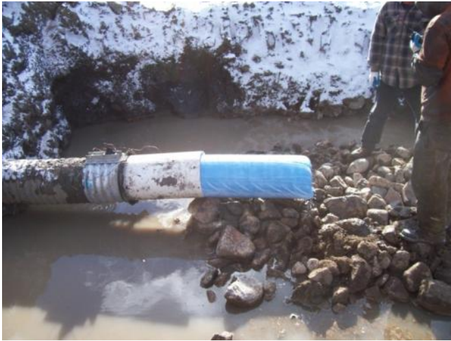
Figure 8 – CIPP after Installation
