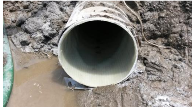
Figure 9 – UV-cured CIPP lining installed inside the existing 12-inch CMP
